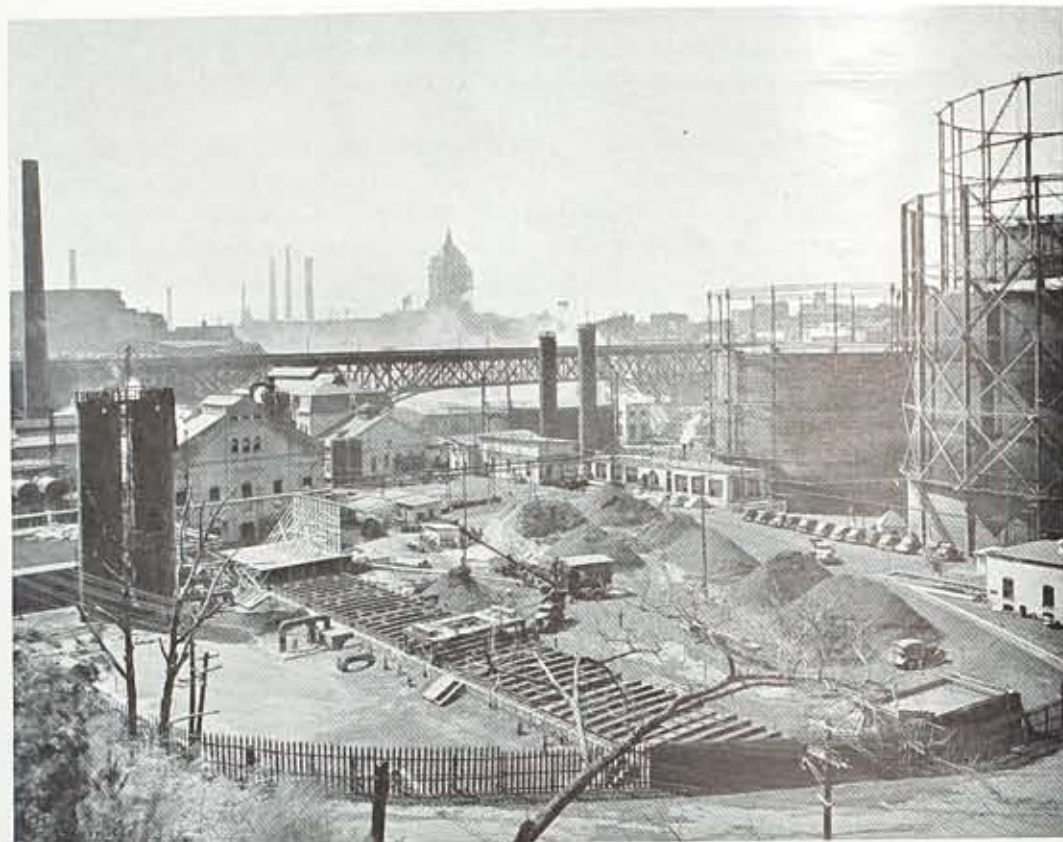
Another view of East Station, looking southward toward Smith Street bridge. In the center are the oxide purifying boxes which remove the final traces of sulphur from the gas, after it has passed through the liquid purifying towers, seen at the left. The two towers in the distance are the light oil scrubbers.
