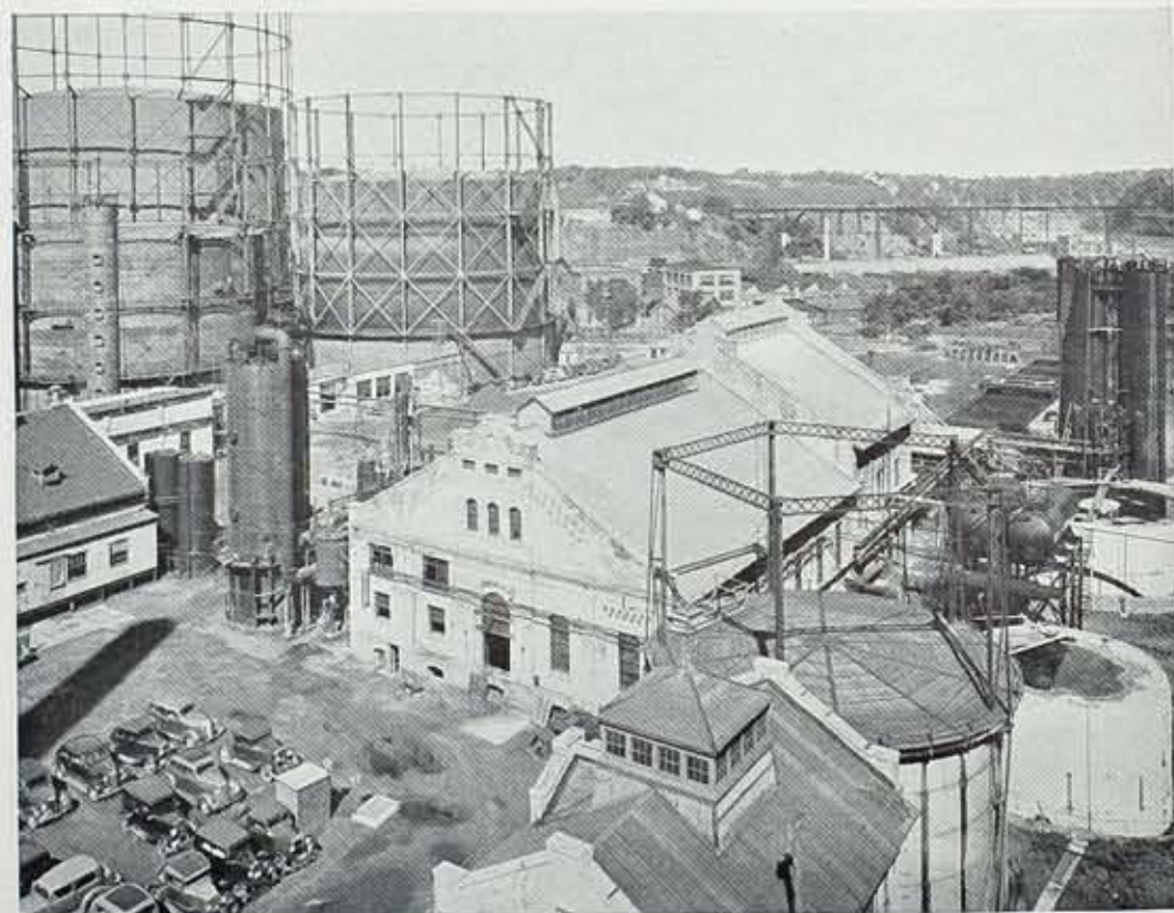
East Station gas manufacturing plant as seen from the eastern end of Smith Street bridge, at the Bausch and Lomb plant. At this plant, gas is purified and metered before entering the gas holders for distribution.
