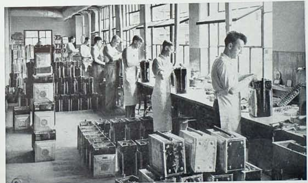
Scene in the Gas Shop, at the Andrews and Front Street offices. Here are inspected, tested, adjusted and repaired, meters and appliances used in homes and industrial plants. From 22,000 to 25,000 gas meters are tested here each year.
