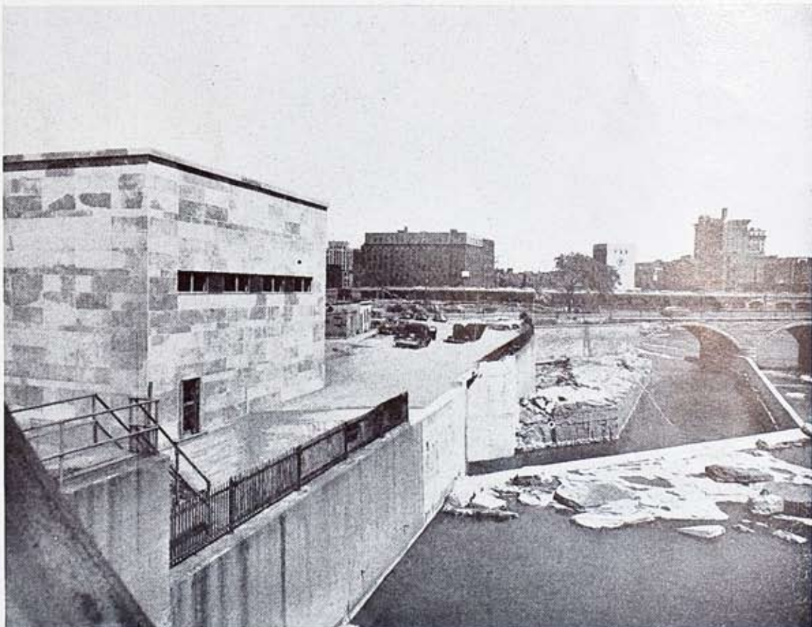
The new R. G. & E. hydro electric station on the river, off Court Street, is nearing completion. It will replace the smaller station which the company, as a good friend and neighbor of the community, relinquished to make land available for the new Memorial Building. The station will have a generating capacity of 3,500 kilowatts.
