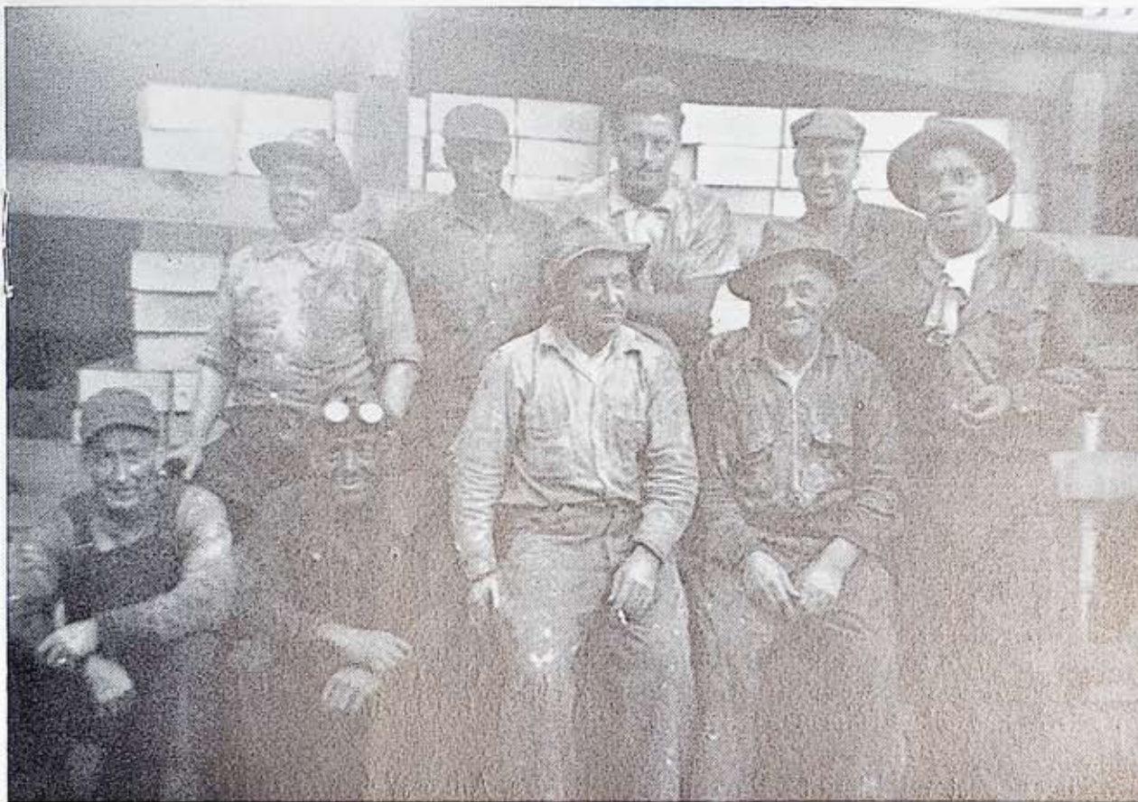
This group of men comprise the majority of a gang that has just completed the repair of the Coke Ovens. The almost constant maintenance of the ovens is one of the main factors in keeping the gas works operating efficiently. One look at the picture will convince anyone that it is not an easy job . . . and it's a HOT detail any time of the year. Front row, left to right: Bill Smith, Bill Major, Tony Mucci, Tony Conversi, and Frank DiMartino. Back row, left to right: Bill Toppetto, Carl Romano, John Ciuffo, and "Pinky" Rosentreter.
