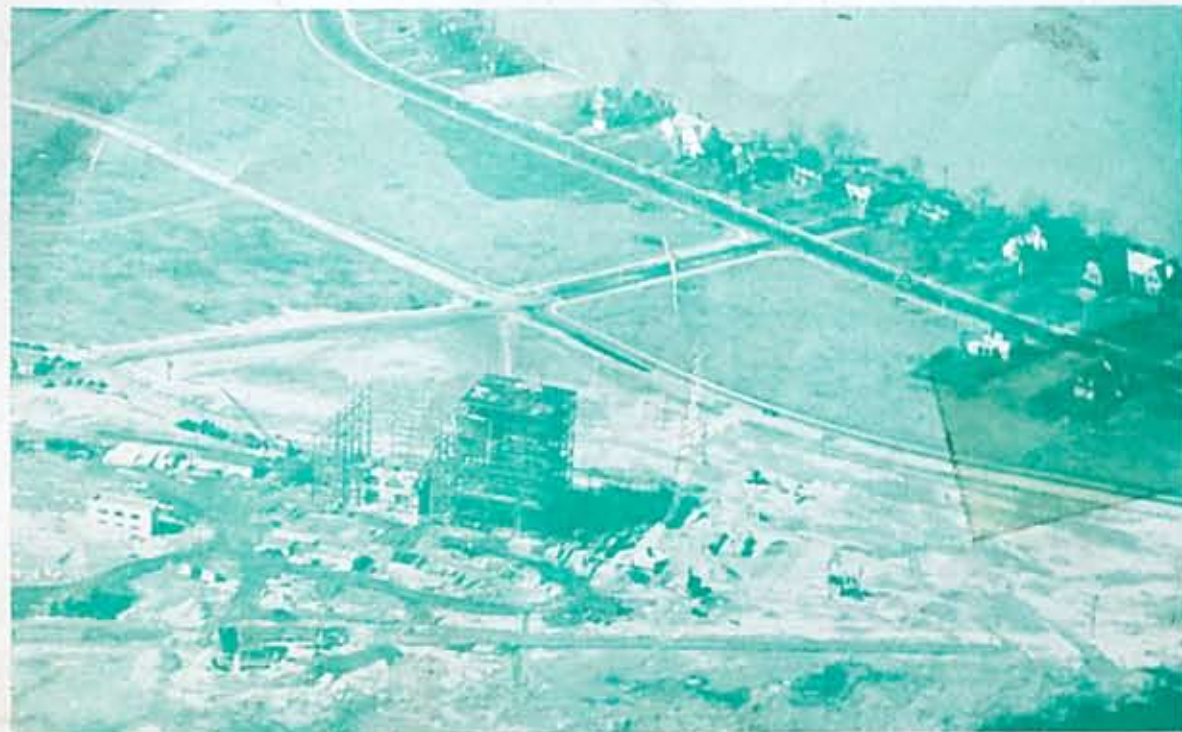
New Lakeside Station in progress of construction
