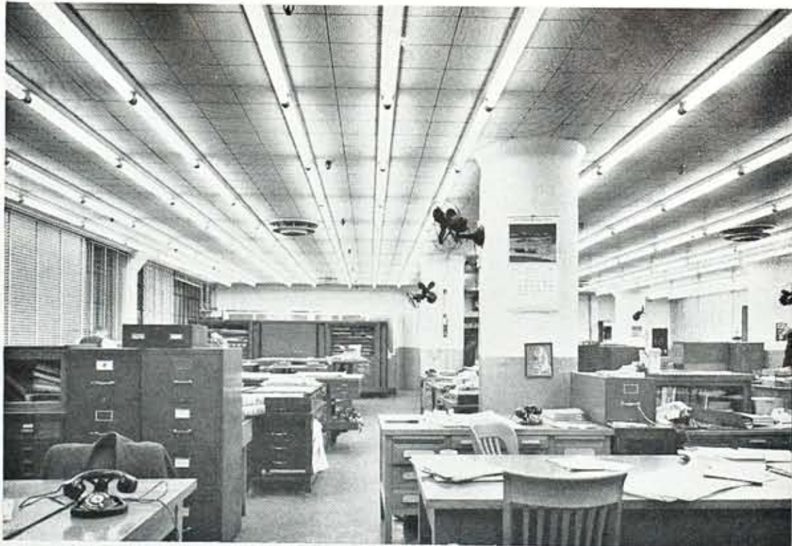
New lighting in the Electric Distribution Engineering office, Front and Andrews, a pioneering application (first of its kind in the United States) of a new low brightness fluorescent lamp, which operates at one-half of its normal power. It provides from 60 to 90 foot-candles of illumination on desk tops and drafting boards. Installation was planned and supervised by Industrial Lighting Department, under lighting engineer Les Twitchell. No employees are shown because the exposure was for about twenty minutes.
