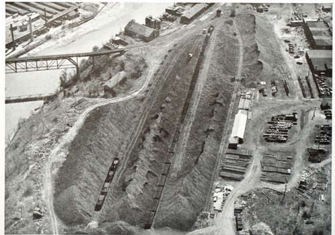
Our reserve coal pile at Ambrose Street which in normal times contains about 100,000 tons of coal for our plants. During the recent coal strike the reserve supply got down to 50,000 tons, or less than 20 days' supply. SEE OTHER COAL PICTURES ON PAGES 12 and 13.
