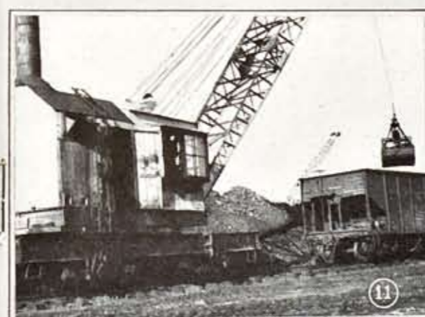
7—Making up a train of coal for R. G. and E. on Charlotte siding. 8—Compacting coal at Ambrose Street to prevent heating. 9—Vista of West Station from State Street coal unloader. 10—One of C. P. Ward's shovels used to load trucks. 11—Locomotive cranes unloading cars at Ambrose Street. 12—Ambrose Street reserve coal pile got pretty flat during the strike.
