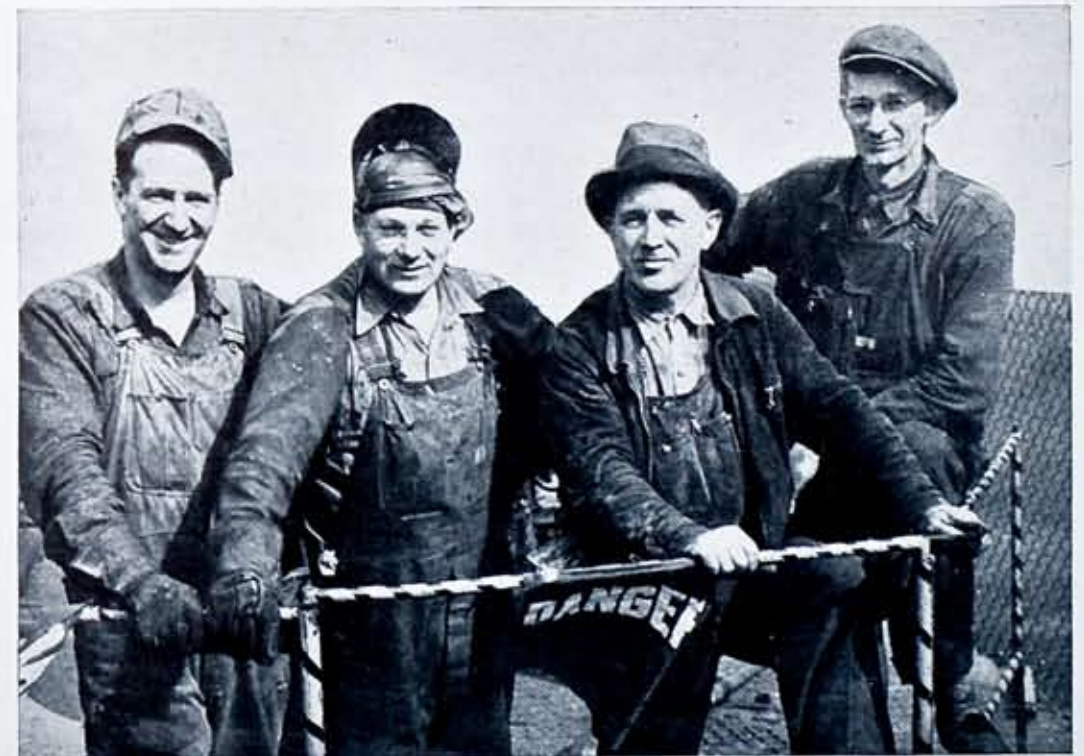
Dick Helfer, Sam Potter, Bill O'Brien and Glenn Pickett come up for a breather. They have been working down in a steam distribution tunnel, where steam mains providing Kodak Office Building and other customers in the State Street sector are being revamped and enlarged.
