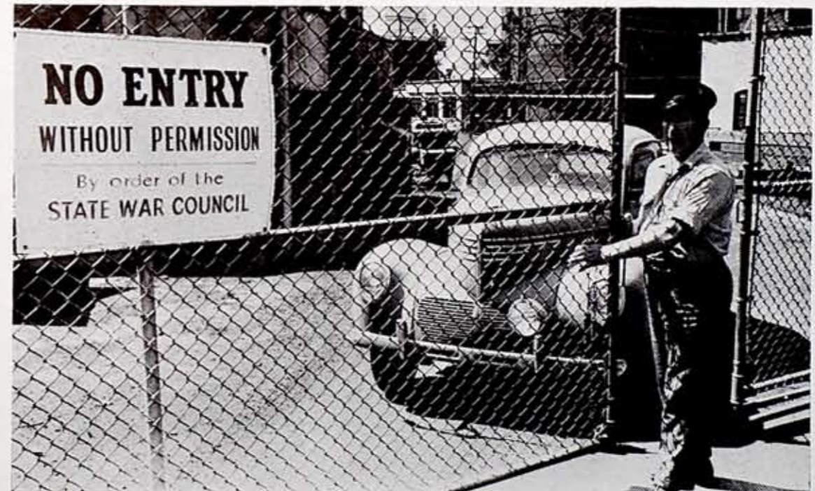
This Company is an essential war plant which provides other war plants with their power, heat, light and steam, without which they could not operate. Shown in picture, Company Guard Bill Magee at West Station Gate.
