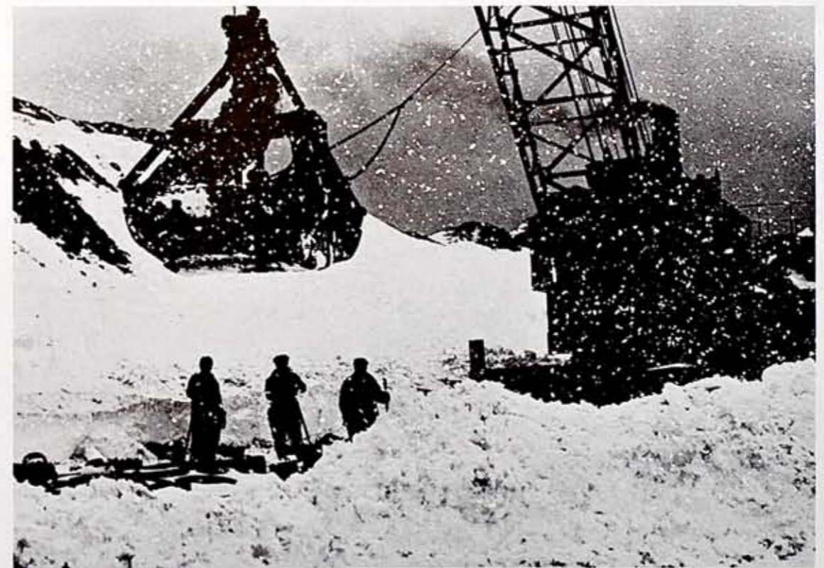
Men take a brief "breather" but the storm keeps right at it, and did so for hour upon hour. Over 70,000 tons of reserve coal are located at Ambrose Street, which is not used until routine methods of transportation and handling are rendered inadequate.
