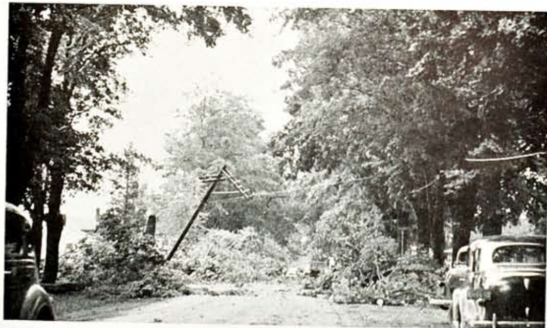
Street in Belmont, showing typical damage done to the fine trees that for years have beautified the village. About one mile of electric lines were torn up and required intensive reconstruction to get back into normal condition.
