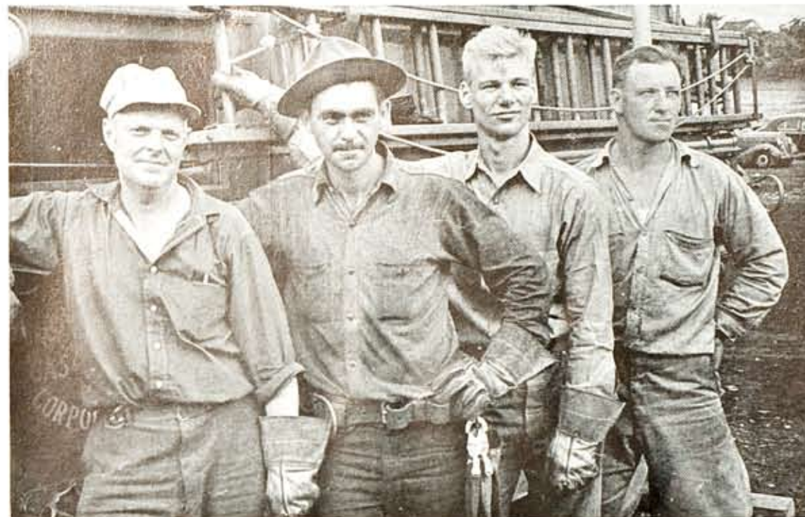
Line foreman Jim Cooper, left, and his men, Albert Connellan, Stanley Hart, and Rudy Kaiser spent many hours arranging lights and electric cables to floodlight the LST 512 shown below during its recent stay in Charlotte Harbor. Thousands of interested sightseers saw and were conducted through this ship.
