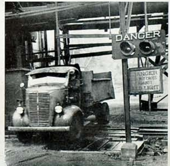
Railway crossing at West Station is well protected with electric safety devices which signal approach of hot coke train.
