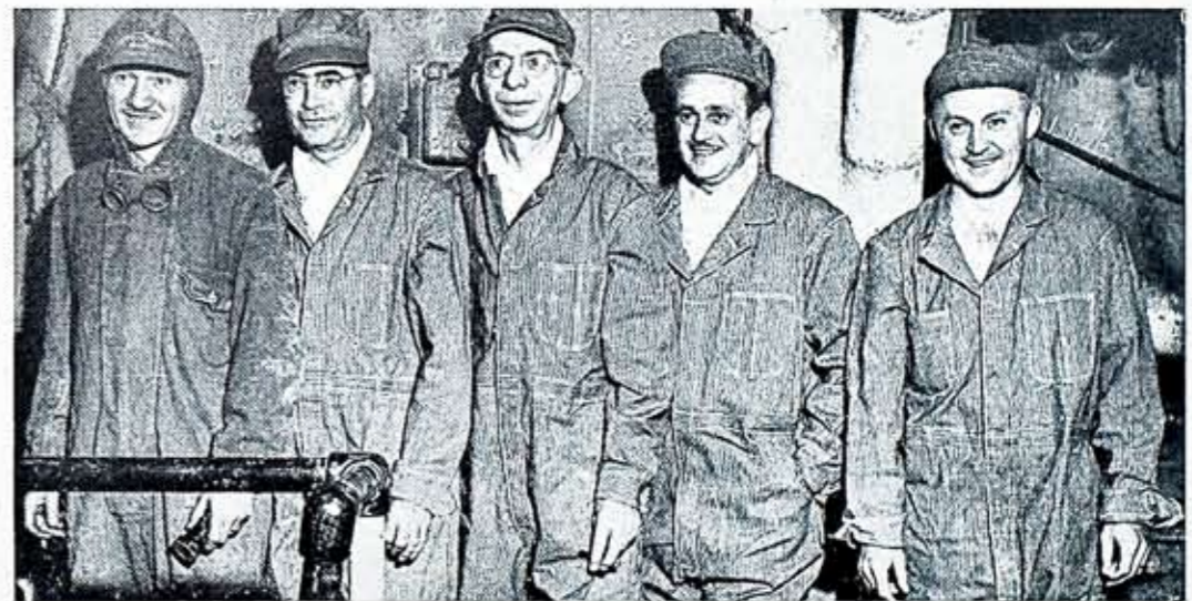
Left to right: "Red" Bert Van Horn, engineer; Walter Consler, Superintendent of the Electric Department; A. C. Veigel, President of the Combustion Engineering Company. Rudy Beckmann, engineer, Combustion Engineering Company and "Cy" Cooley, engineer, Station Three, just before they entered No. 1 boiler at Station Three on an inspection trip.
