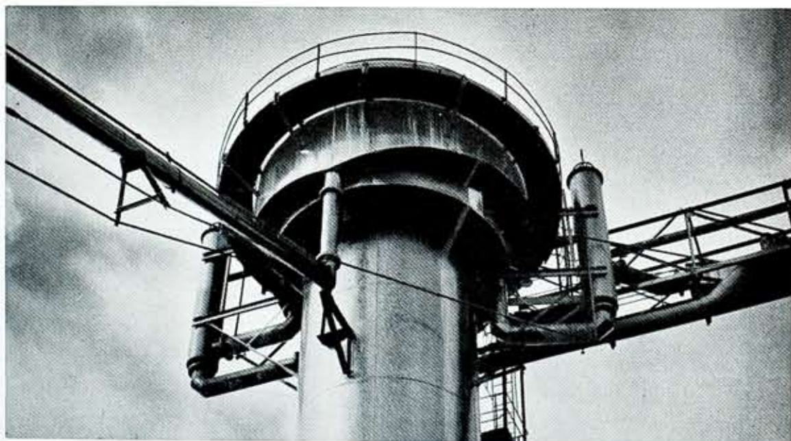
Tower of large light oil scrubber installed at East Station during 1937. It operates in parallel with the original scrubber there.
