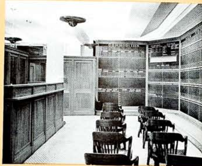
Board Room lighting, A. J. Wright investment house.
