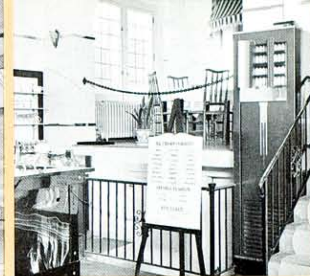
Unit gas heater (in cabinet) at Love's.
