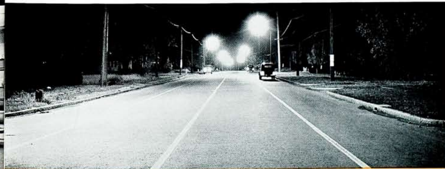
St. Paul Boulevard, Rochester, N. Y., one of the finest lighted thoroughfares embodying modern safety lighting. During the past year these Sodium Vapor lights resulted in effectively reducing loss of life due to motor vehicle accidents. It is called the "path of gold."
