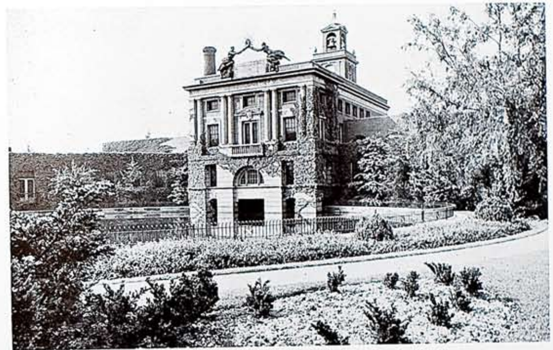
View of the beautiful Institute building, where the chorus sang, a building literally filled with interesting exhibits relating to electrical progress.
