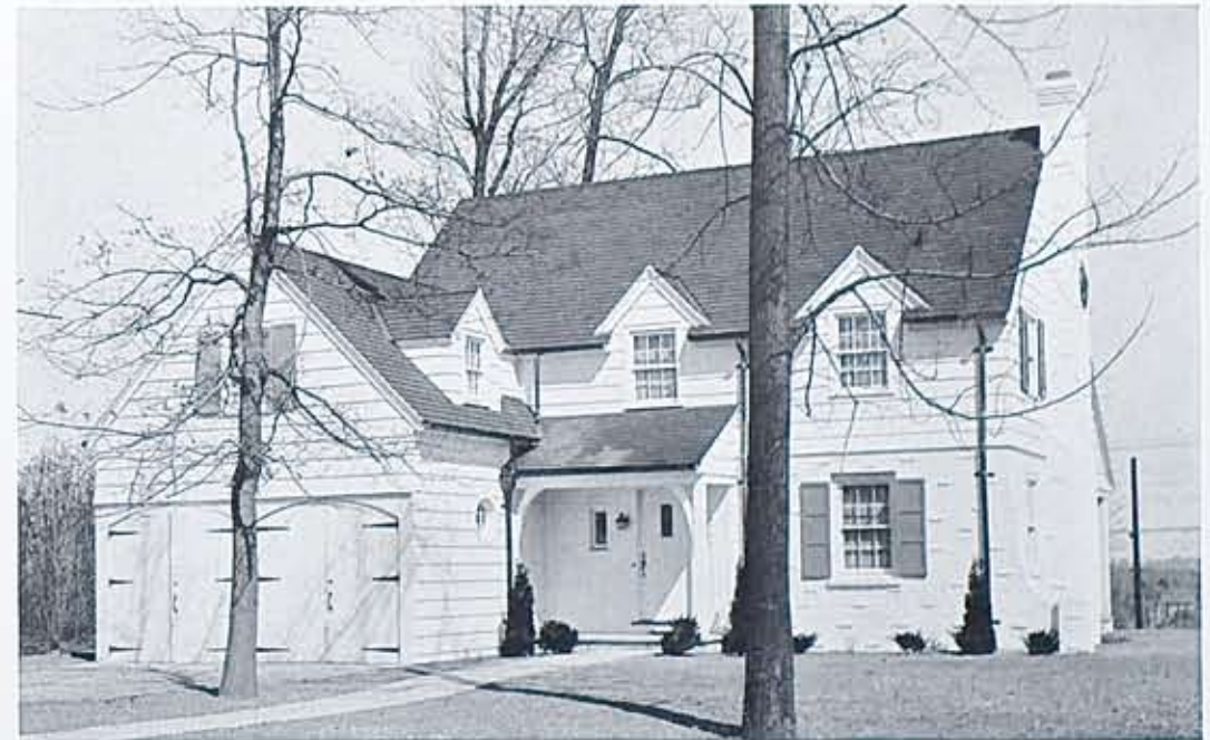
The Windsor model home, one of Rochester's first gas homes to be thus featured. It is equipped with gas home heating, Electrolux (gas) refrigeration, automatic gas water heating, has a gas disposal unit besides all of the modern electric appliances of the day. The cover picture shows a corner in the kitchen, where the 1937 Electrolux holds forth.
