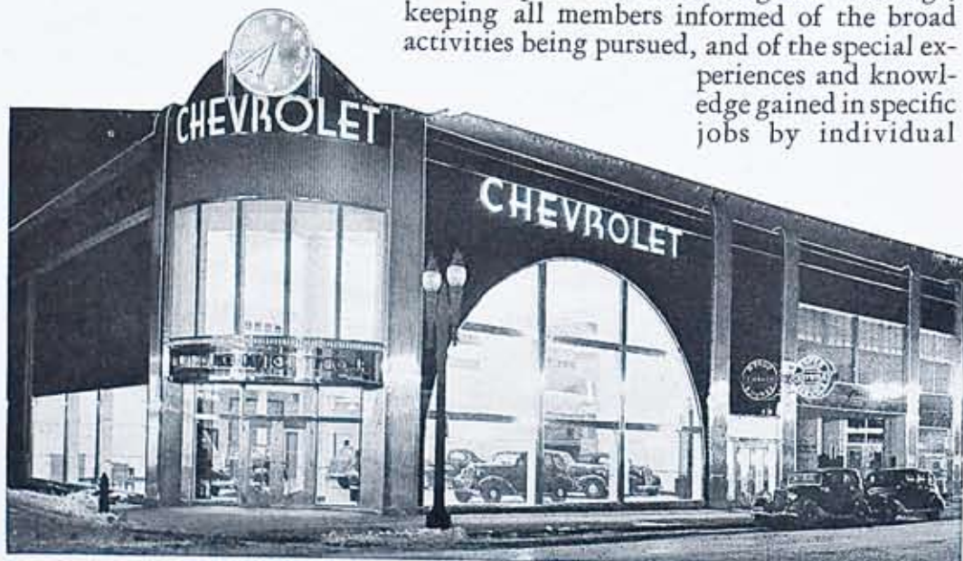
Central Chevrolet Building, East Avenue. The Industrial Department cooperated with Mr. Harry Fincher in the planning and designing of this fine lighting job. Electric signs are here used as a unit in the building design.
