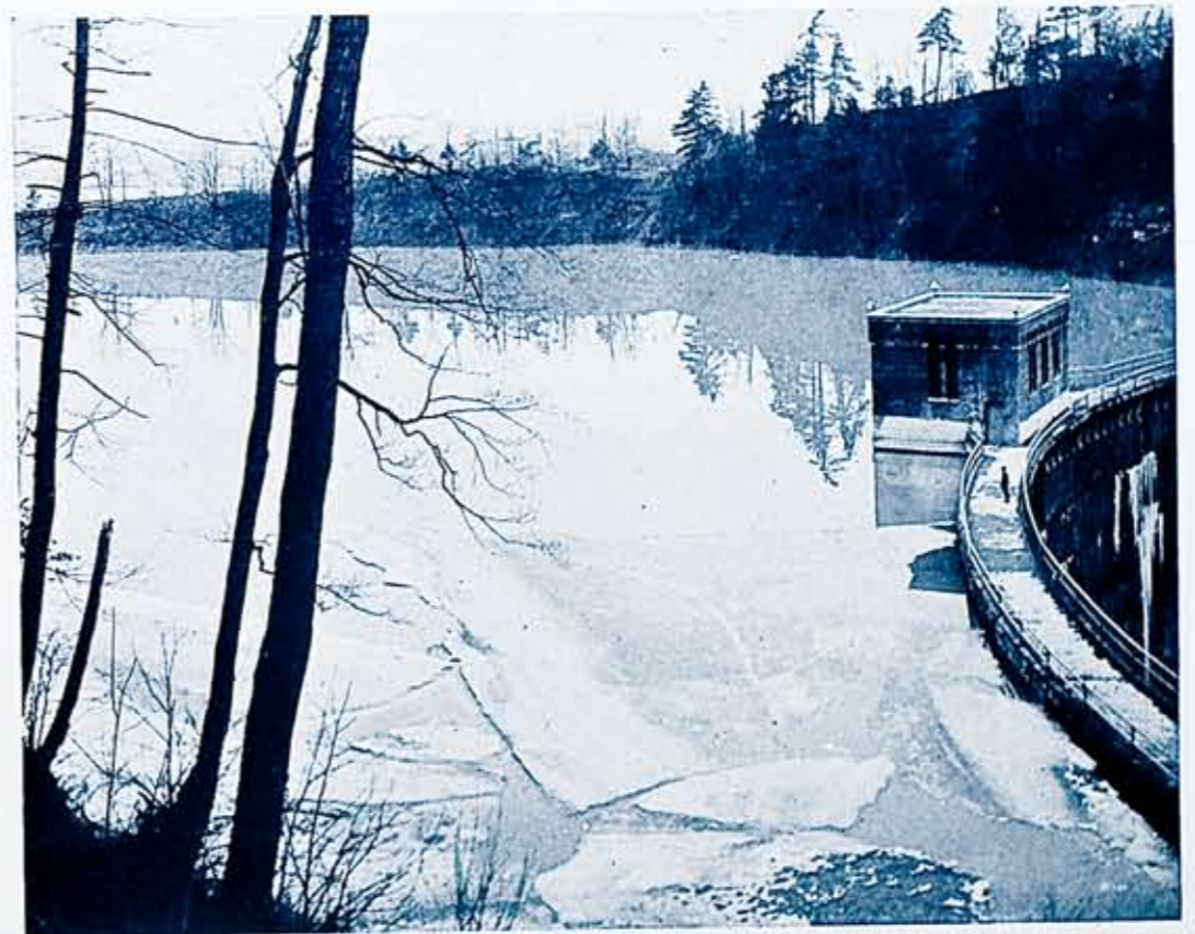
Top: Upper side of the Caneadea Dam in spring time when the water is high. This impounding of water helps as a flood control measure and water is dispatched from here to be used in the hydroelectric plants at Rochester. Bottom: Scene at the dam when the ice was melting in early spring.
