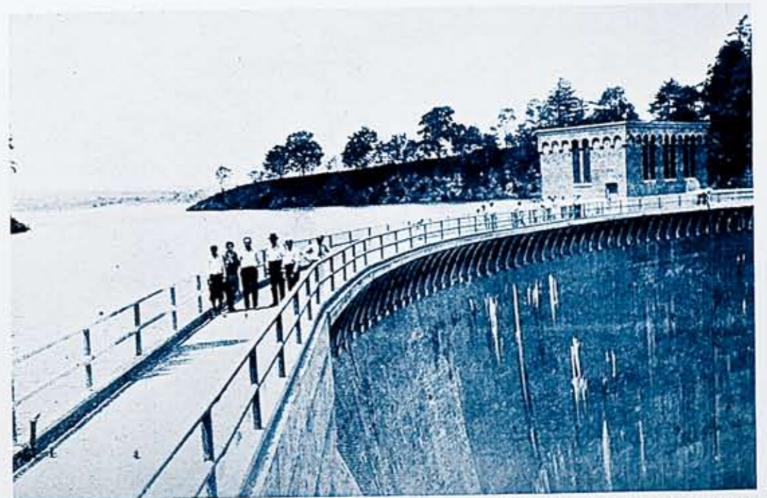
Section of lower side of the Caneadea Dam, across the top of which there is a walk from which delightful views may be had up and down stream.
