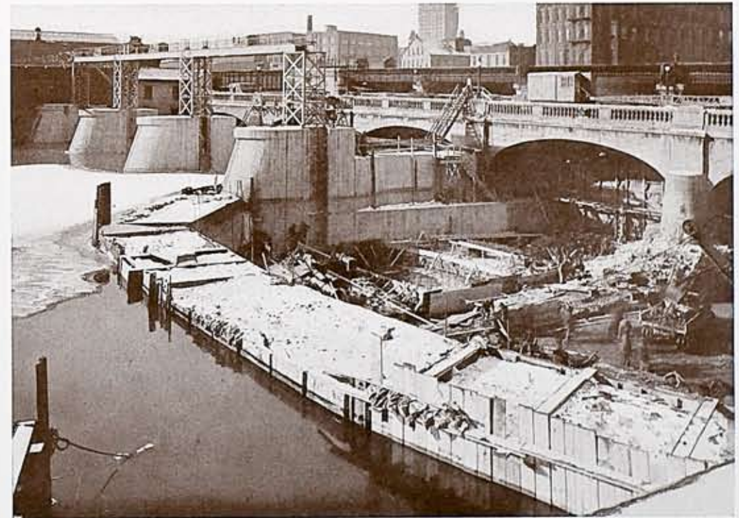
This view shows the job as it appeared about December 8, 1936. The first three gates were then completed and the waters of the Genesee River have been held back by cofferdams as work progresses on the last three gates.
