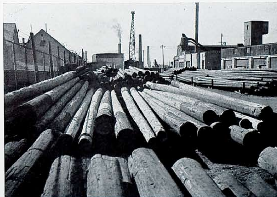
Some poles. These wooden poles in the Company pole yard, Atlantic Avenue and Leighton Avenue, represent a large investment when it is considered that about 10,000 wooden poles were used last year mostly in rural extension work. About seventeen poles are used to the mile, and the largest poles cost about $50. The purchasing department not only has the purchasing responsibilities of the Company, but also makes analyses of requirements for the present and future. In these days of rising prices, this is an important, responsible activity.
