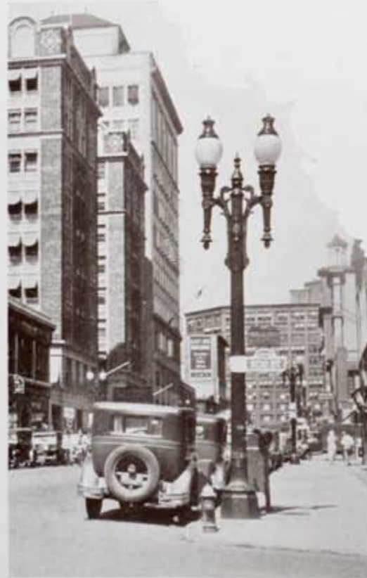
Type of modern street lighting on East Avenue, fed from underground cable, making for more beautiful and safer streets. A total of 27,628 street lamps serve Rochester, one of the best lighted cities in the country.
