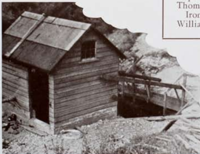
Pump house, Barker farm. Water is found in abundance at the base of this old gravel bed. A small electric line was built by Mr. Barker to this pump house to supply power.
