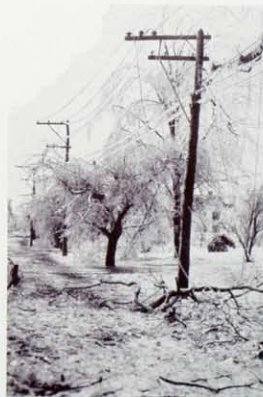
Where adequate line construction helped to save the day for electric service. Among the great constructive factors in restoring service was the group of tree-trimmers who mopped up nature's confusion for line gangs.
