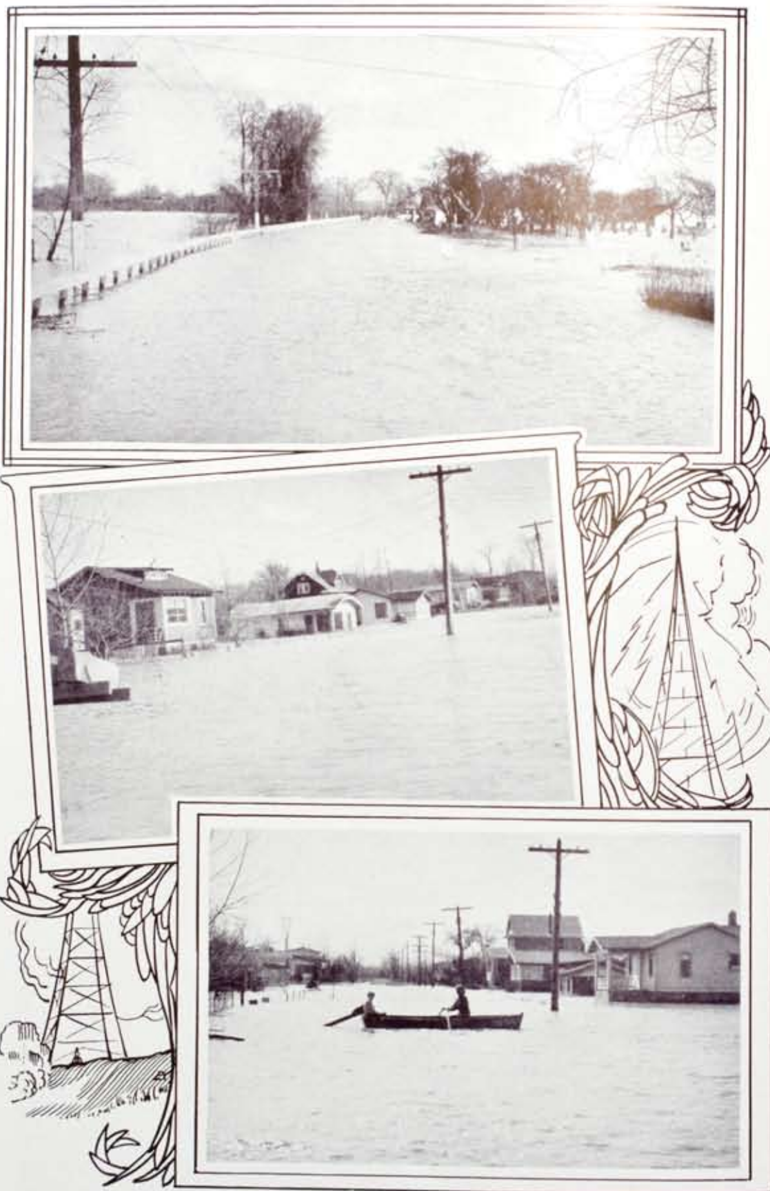
A few flood pictures taken by Arthur Underwood. Top, where the Genesee River took liberties with the River Road. Wires high up on sturdy poles gave service as usual, although folks had to get food in rowboats. Center, and bottom, along Idle Lane, where the old song "River stay away from my door" was of little benefit in keeping off the advances of a Genesee on a spree.
