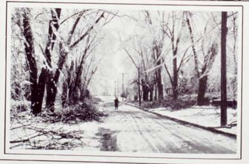
The sleet storm in Canandaigua, N. Y. Top, pole down on Chapin Street, March 18, where there was a chance for some real "fireworks" tying guy wire on 33,000-volt transmission line from Rochester, March 17. The Rochester line was cut after breakfast was served at the U. S. Veterans Hospital, 9:25 A.M. Telephone lines are underneath. Bottom, beauty and the beast, on Park Street. The Rochester line held throughout all the trouble, a great "break" for Phil Thomas and his men as well as Canandaigua and vicinity.
