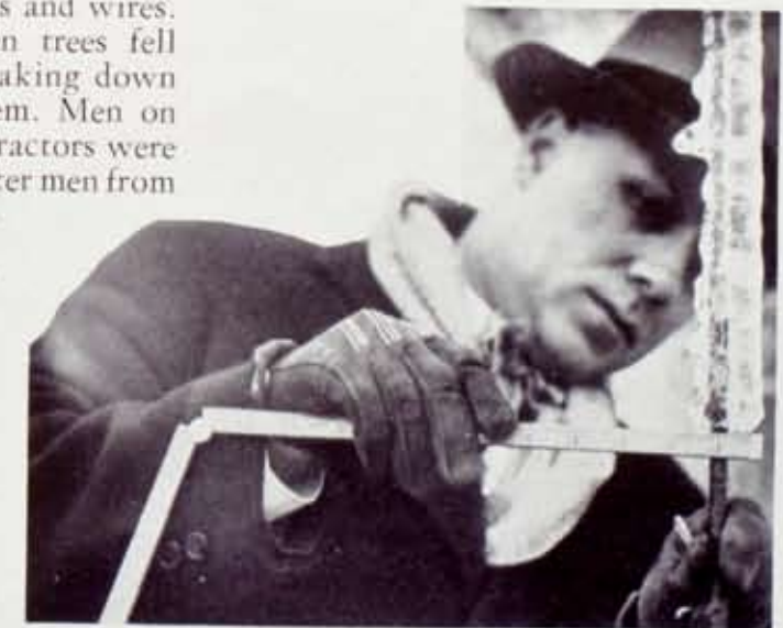
One morning when all Nature was a huge refrigerating machine or ice-maker, Schuyler Baldwin, Canandaigua, measuring the accumulation on a power wire.
