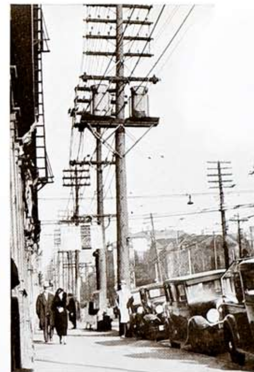
Toronto street scene showing overhead distribution system and transformers mounted on poles, with small lighting units, or lamps barely noticeable.
