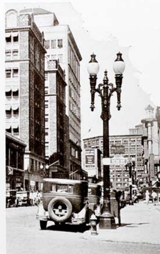
Scene on East Avenue near the Rochester Club, Rochester, N. Y., showing ornamental lighting poles carrying lamps served by underground distribution system.
