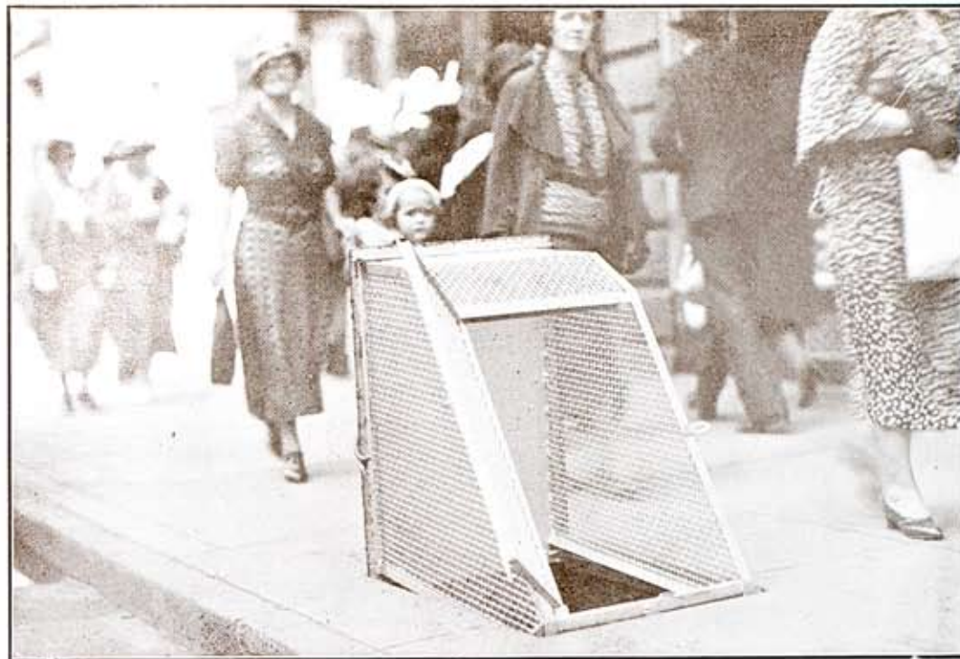
Safety First. "Help us to Prevent Accidents" is still a good slogan. The special manhole safety entrance shown above as installed on the Clinton Avenue vault helps to do just this. When men are working in this vault, red and white safety flags are hung from the safety entrance.
