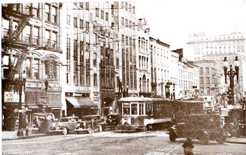
Typical downtown Rochester view showing a pleasing absence of overhead lines or poles or transformers. The usual construction here is underground 4,150-volt feeders and distribution transformers and secondaries.
