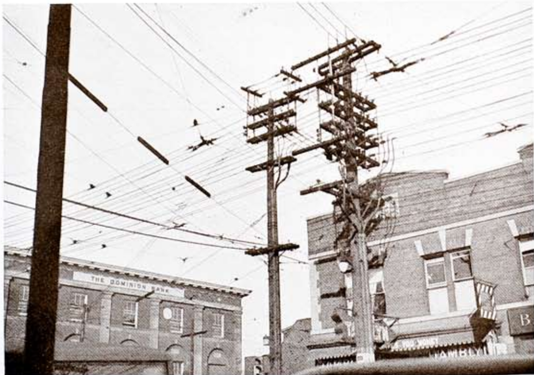
Scene typical of Toronto's distribution system, with overhead poles and wires which are especially noticeable to persons who have lived for some years in a city where no such array of physical equipment clutters the downtown area. Underground construction costs a lot more, but most persons think it is well worth it in factors of safety and service.
