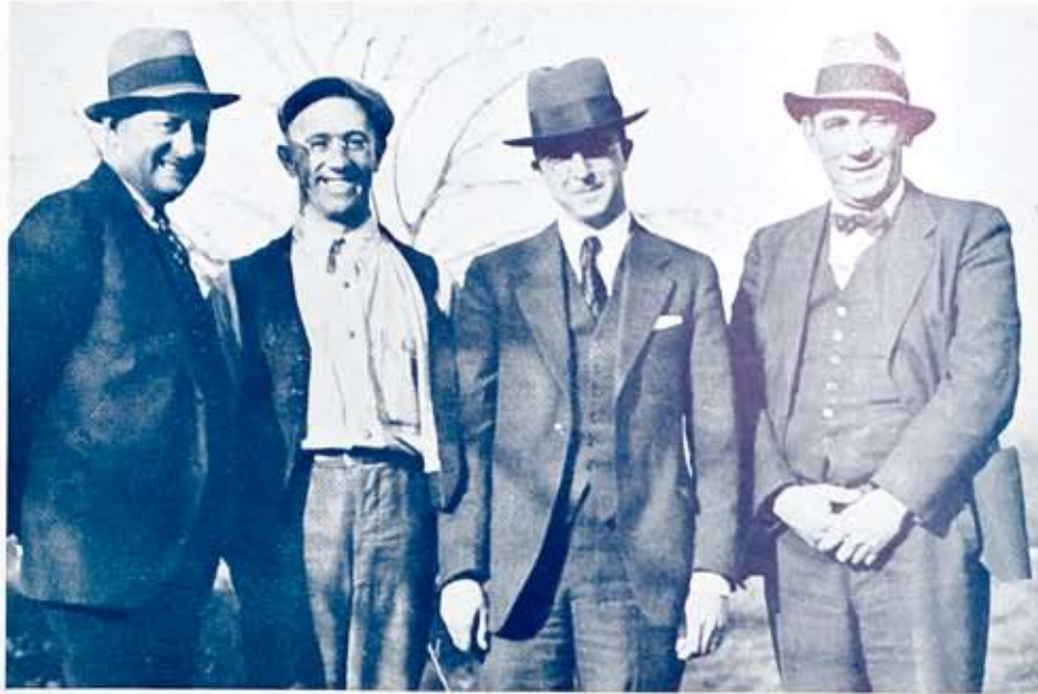
Messrs Ralph Mason, Abram Moll, Lucas Caple and Fred Wood, who installed the electric heating apparatus shown in center of picture below. Mr. Mason and Mr. Wood are from the Lake Shore Division of the Company, Mr. Caple being a member of the Industrial Department of Rochester.
