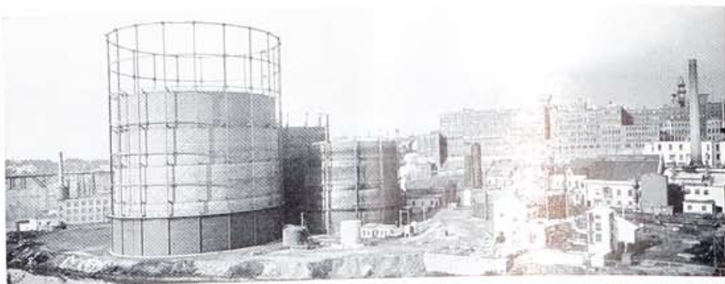
Part of Rochester's fuel bin, at East Station, along the east side of the Genesee River, below the Bausch and Lomb plant, from which gas is pumped to customer's premises. The gas holders at this point are capable of storing over 8,000,000 cubic feet of gas, or about one day's supply for Rochester under normal winter demand.
