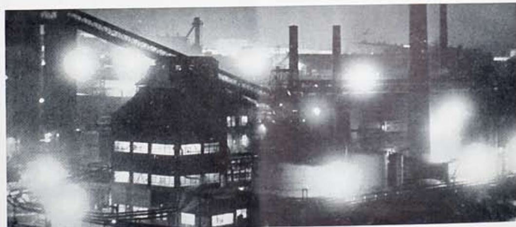
Night view of West Station gas works. The gas-making process is continuous, night and day, throughout the year and provides uninterrupted service for Rochester homes and industries. About 215 men are employed in this large plant, in three daily shifts.
