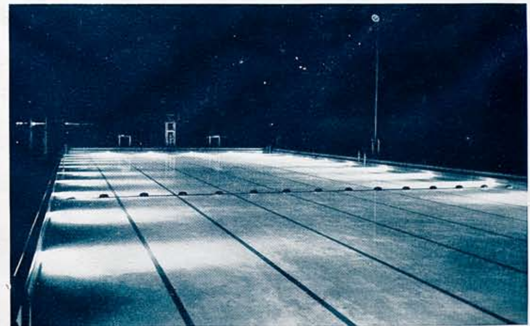
One of the pools showing the under-water lighting turned on, with the overhead lighting off, to show the intensity of the under-water illumination which is sufficient to follow a swimmer from one end of the tank to the other.
