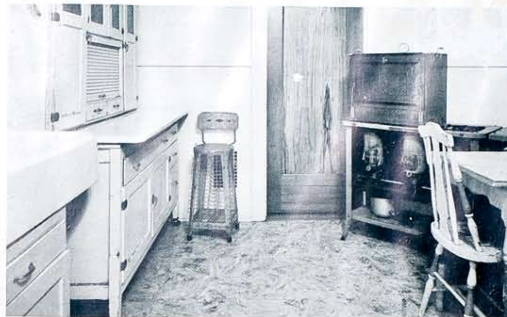
Kitchen of a rural home which recently installed an electric range and an electric refrigerator (before the transformation was made, including the redesigning of the cupboards).
