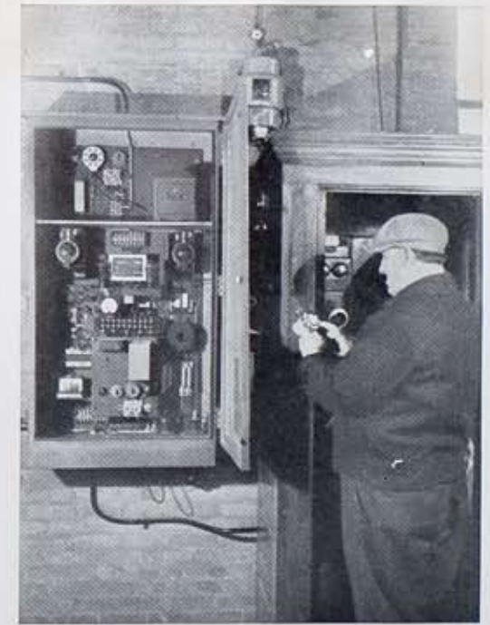
Mr. Edward Parmelee dialing for a switching operation at Carrier Current set.
