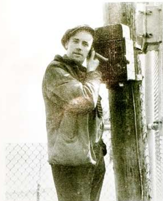
Lineman Hamilton Bailey telephoning from the Company's private telephone box at substation No. 43. Trouble men keep in constant telephonic communication with the Line Operation Department, so that they may be dispatched without delay to clear up trouble of an emergency nature.
