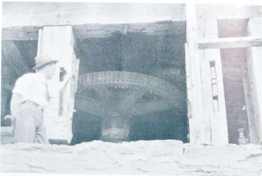
Note the heavy construction of this old mill and the wooden wheel, even the gears of which were wooden. Mr. Caple is seen examining the construction of this old mill's equipment.
