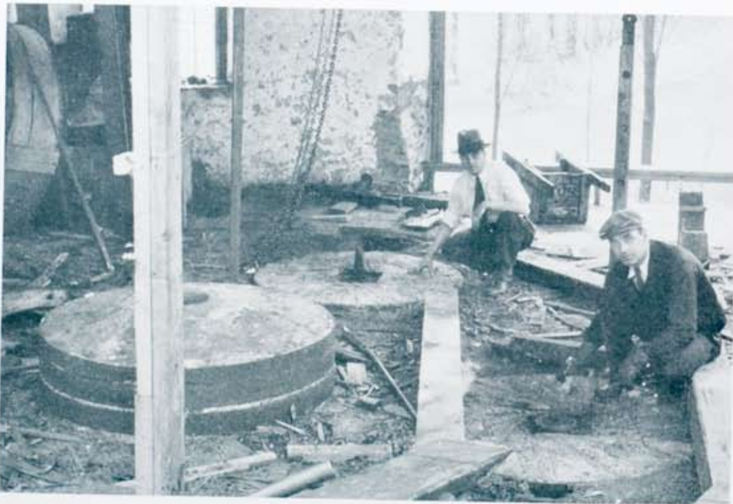
The three mill stones as they were originally located in the old mill. As they were turned, the grain was ground and shoved outward to the stones edge from where it fell downward, to the floor below for bagging. At the left is seen a pair of stones, both the upper and lower stones being in place.
