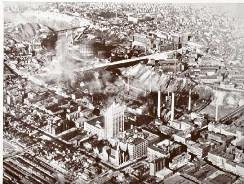
Aeroplane view of a section of Rochester showing the Genesee Gorge between Platt Street bridge and the N. Y. C. Railroad bridge, with Smith Street bridge near the center. Kodak office building is in the center foreground; east of it are to be seen the chimneys of Station 5 and the West Station Gas manufacturing plant. Below Smith Street bridge are the gas holders of East Station, the Bausch and Lomb Company.
