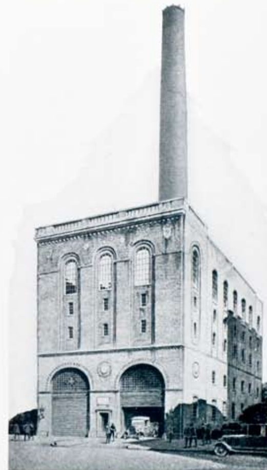
The commercial district heating plant Station 8, Lawn Street at the rear of the R. G. and E. Bldg. This modern powdered coal steam generating plant serves all of the new buildings and many other customers in its district in the downtown section of Rochester.
