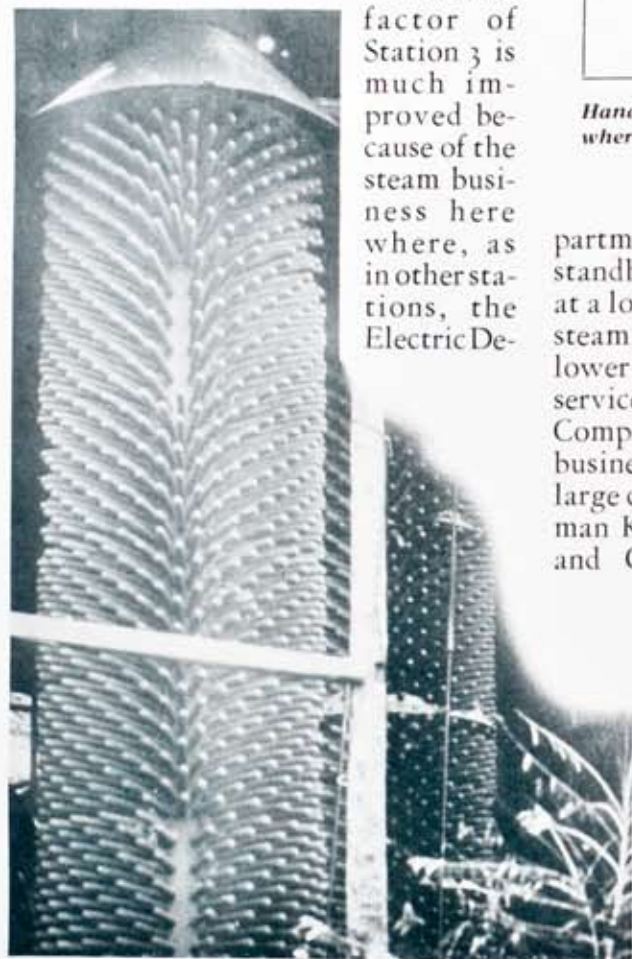
"Porcupine" boilers formerly used at old Station 2 on the Genesee River flats near Platt Street. This station had eleven of these 500-horsepower, 175-pound pressure boilers. Installed in 1892, they were hand-fired through three doors in the cylindrical base.
