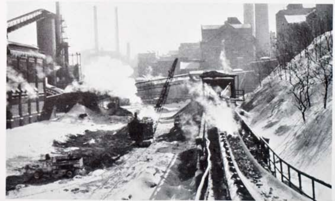
Section of West Station Gas Manufacturing Plant which presented a bleak, frigid aspect during the coldest "spell" of weather Rochester has ever had. At the right is shown a long section of the conveyor belts, of which there is a total of over one mile in the plant.
