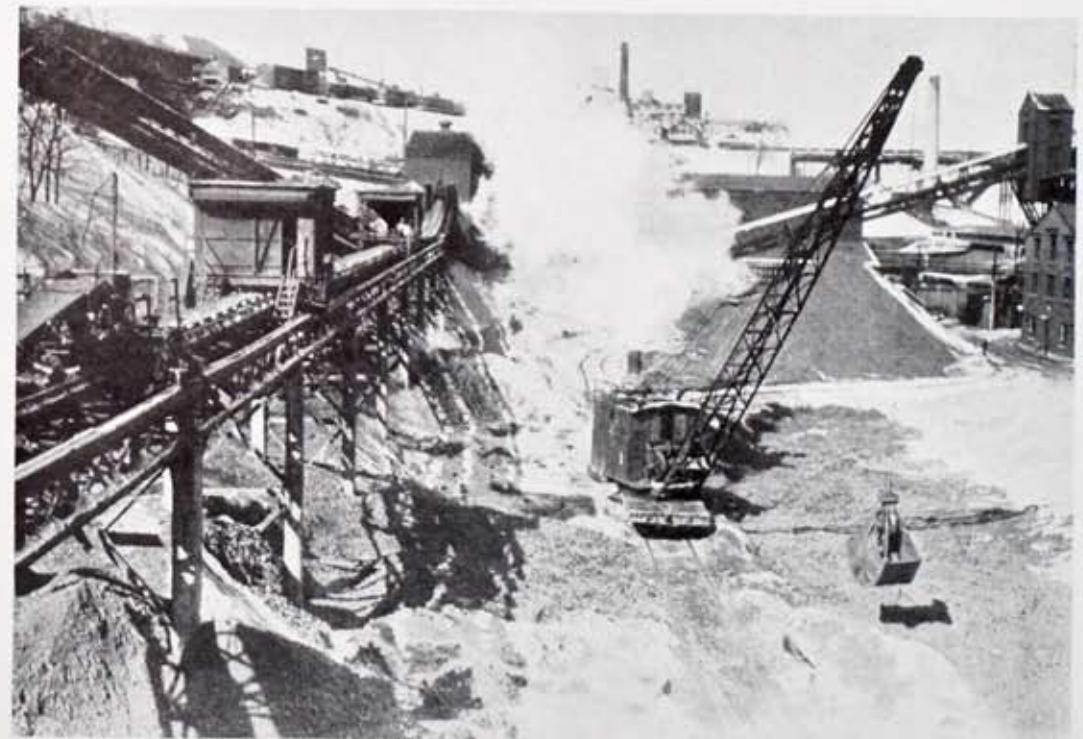
View of a section of East Station showing another long stretch of conveyor belts at the left. The steam shovel picks up the coke in the yard and deposits it on a belt which transports it to the crusher house, in the left distance.
