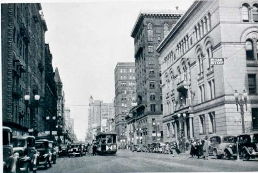
This view of Main Street corresponds to the one shown on the opposite page, but was taken a half-century later. It shows West Main Street as it is today, free from overhead lines. Rochester perhaps has more underground electric lines than any other city of its size and class in this country.
