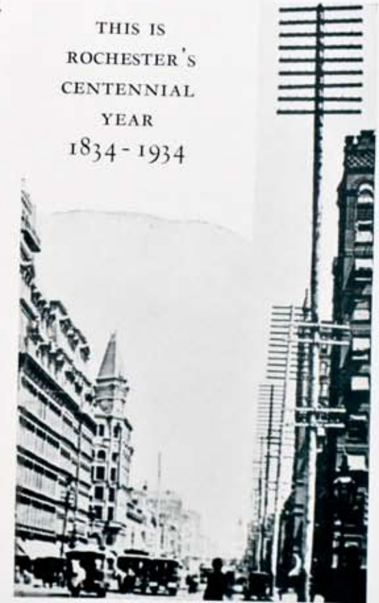
Looking east toward the "Four Corners" in the days when 75-foot poles were not uncommon and when all lines were of the overhead type. Today all of Rochester's downtown section is served by underground lines.
