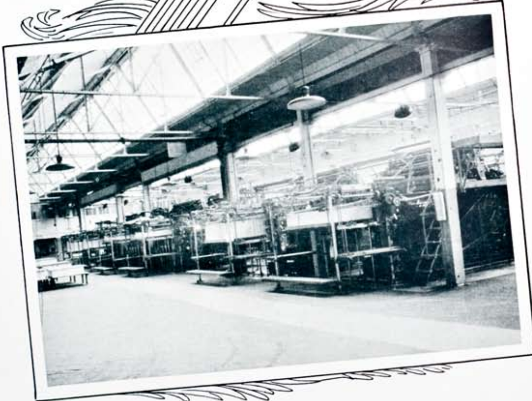
Top, Air conditioning at the Eastman Kodak Company is absolutely necessary to maintain constant conditions of temperature and moisture and to keep dust out of the atmosphere. It is a great aid in film coating, drying and paper making. Bottom, this room at the Stecher Lithographing Company is air conditioned to keep paper from stretching and of exactly the same size between multiple runs, for proper register.
