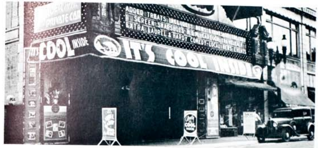
Rochester Theatre advertises its ability to keep people cool and comfortable on hot days. Air conditioning is found to be a box office booster in the amusement world, and a business builder generally in other lines. The public appreciates any effort made to contribute to their comfort.
