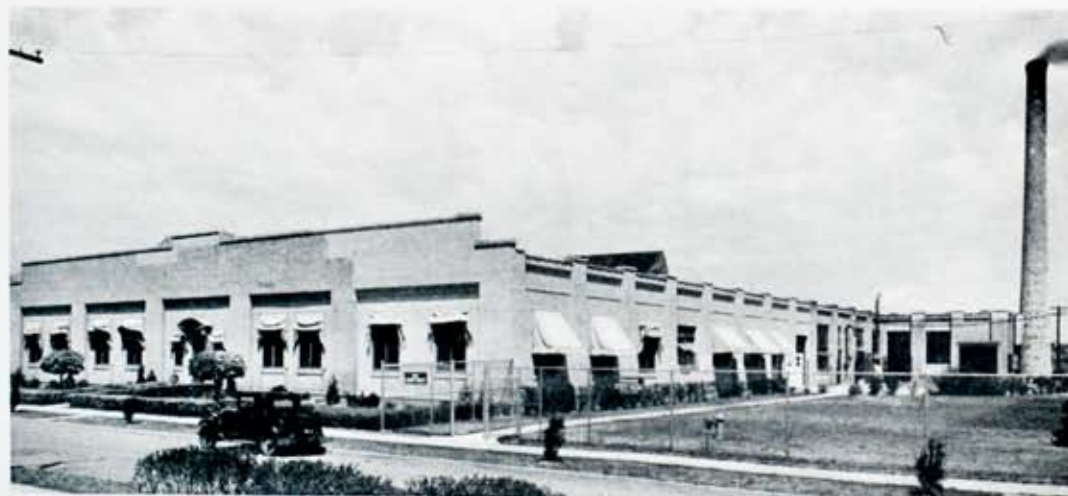
Plant of The Haloid Company, manufacturers of photographic papers. Here air conditioning is used to maintain the exacting temperature conditions required in applying emulsion to photographic papers and drying it within the requirements of very special conditions.
