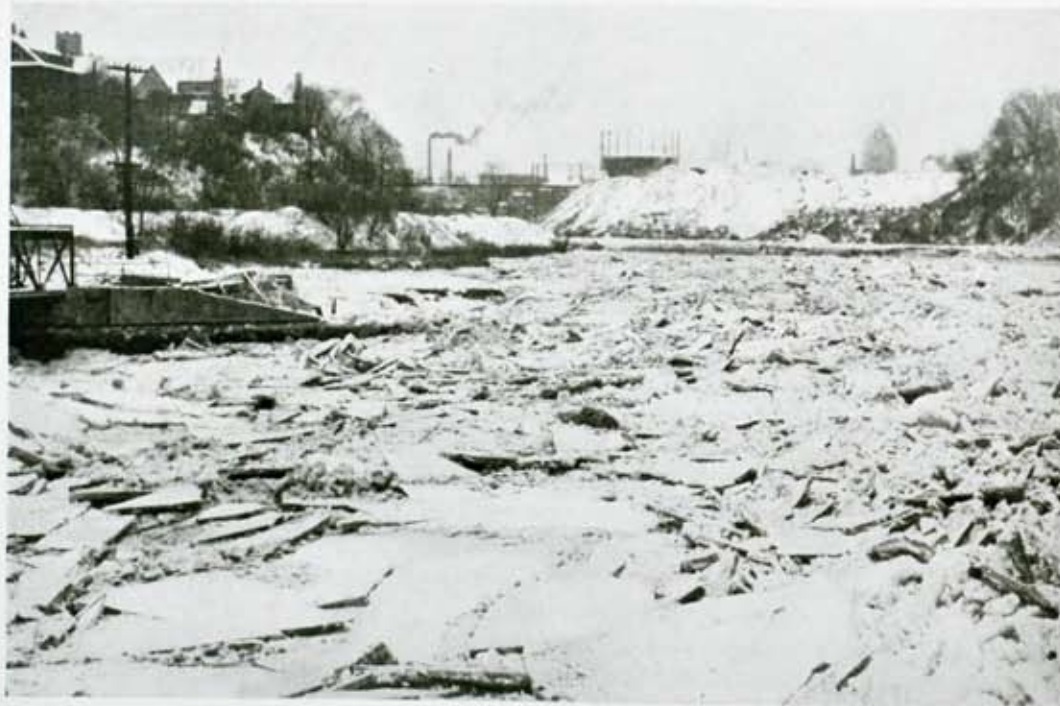
Looking south from the intake house at the Headgates of Station Five, showing east side of the Genesee River pond packed with ice. Ice in this pond usually goes out before the upper river ice arrives. This year, it was thick and well anchored to the shore and pond bottom, therefore comprising one of the reasons for the ice jam, which formed just beyond the curve in the river.
