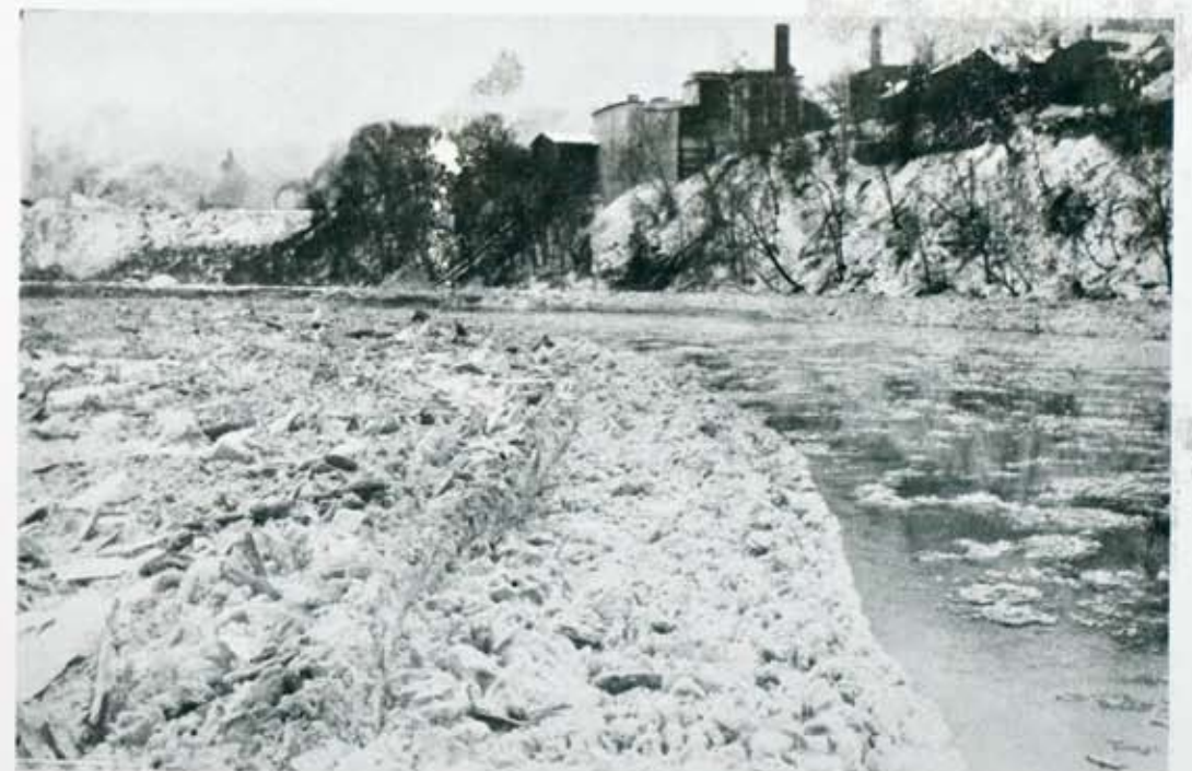
Companion picture to one on opposite page, showing west half of the river just after the ice jam was broken and the flow ice began to come down stream. Much of this ice jammed the intake racks, preventing water entering the huge tunnel waiting to conduct it to Station 5, at the Lower Falls.
