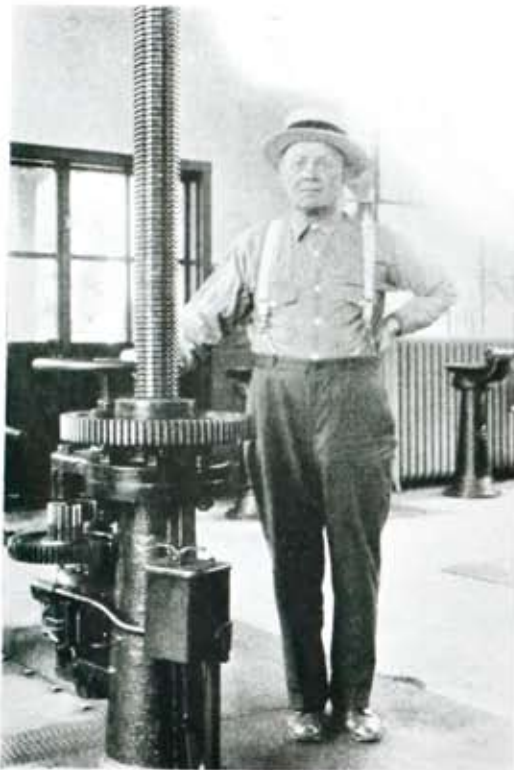
Mr. Andrew E. Johnson at one of the sector gate controls which operate the mechanism which opens the gates when it is desired to spill water over the dam.
