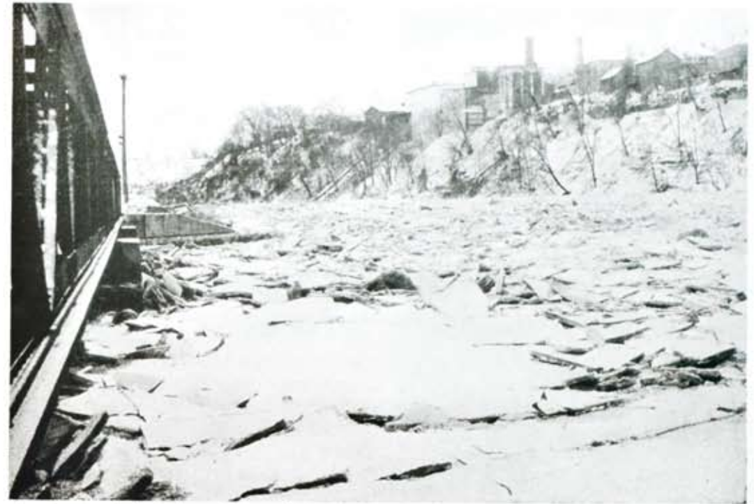
Another view of the ice jammed in at the top of the sector gates, shown below, after the ice jam upstream gave way and released the tons of pent up water which rushed downstream like an avalanche. An all-time high water mark was set upstream, north of the Upper Falls, the water reaching a height of sixteen feet at Station 2 where it began rushing into the station doors and windows.
