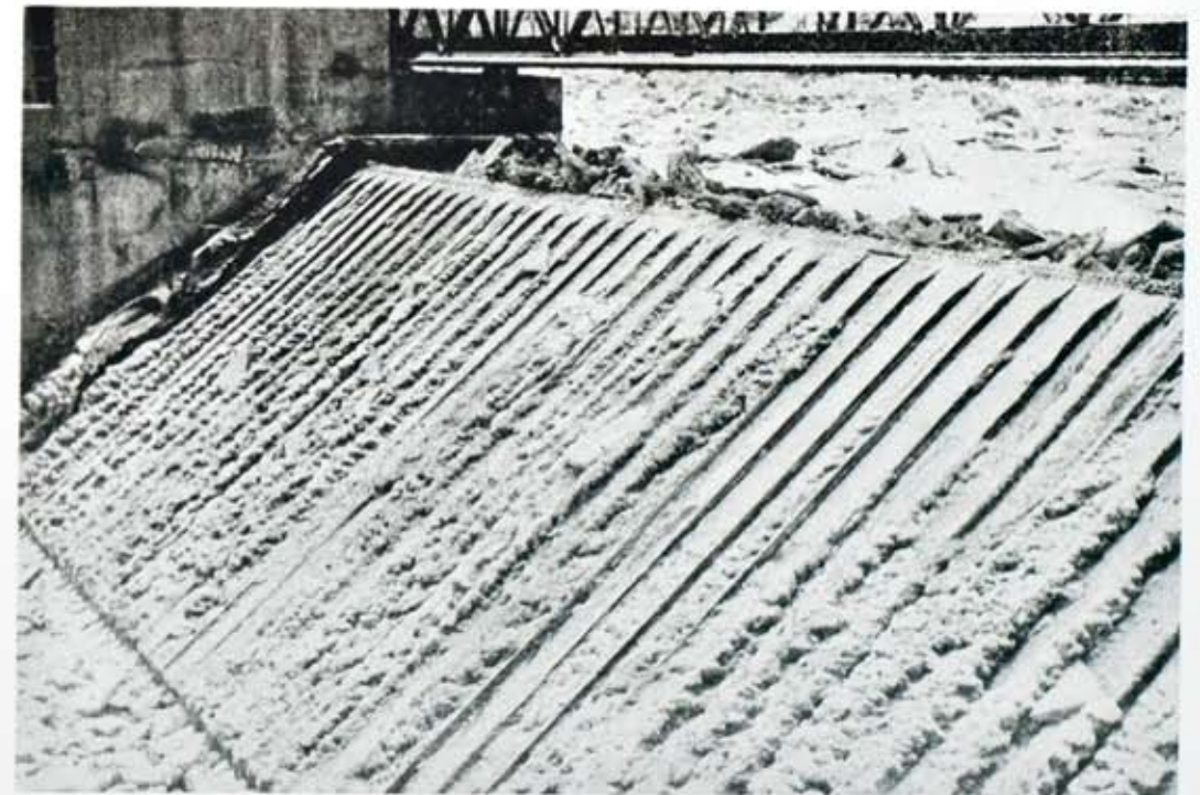
One of the Station Five Headgate sector gates which was opened soon after this picture was taken to help release the flood water and thus help to break the huge ice jam above. Old Man River kept scores of employees busy doping out the proper "next move". It was not unlike a game of chess, but eventually, the river lost.
