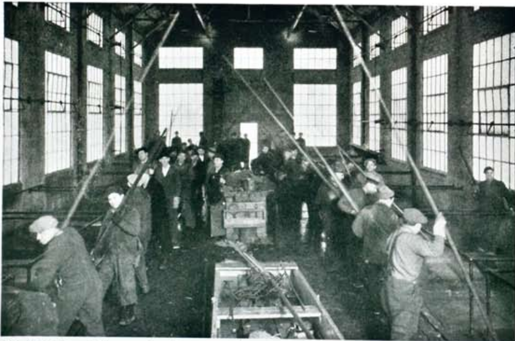
The Headgates rack house, where Company employees from various departments were pressed into service to free the tunnel intake racks. With long-handled grappling hooks, these men are shown hooking out the tons of ice and debris collected in the racks at either side of the long building, thus making it possible for water again to enter the intake to the huge underground tunnel which conducts it 1,500 feet underground to the turbines at Station Five.
