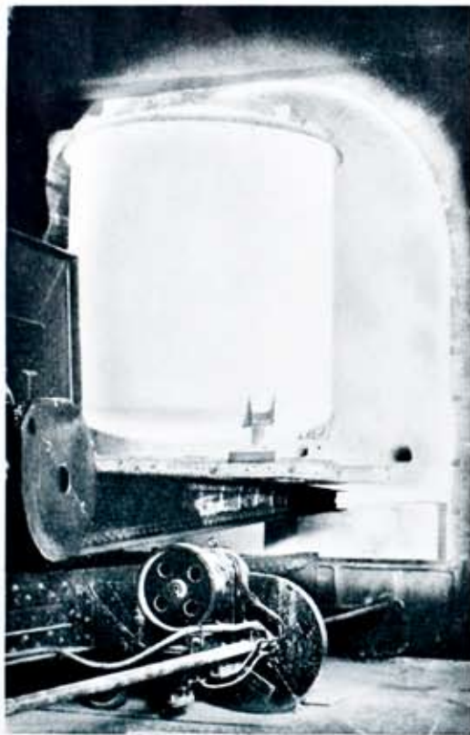
Pfaudler glass enamel is fused into steel base of vessels in large enameling furnaces such as this one at temperatures averaging 1800° F. Photo shows vessel just as it was being removed from furnace by an electric charging machine.
