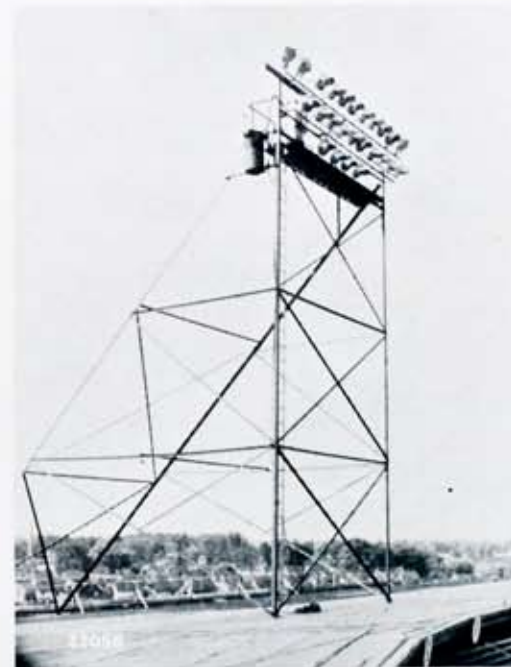
Left: Steel tower on top of grandstand, showing its transformer, and the flood lights directed at the infield. A similar tower is at the other end of the grandstand.
