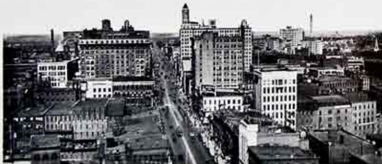
With more than 300 private boiler plants and their smoking chimneys discontinued in favor of the Company's steam service, the effect upon Rochester's skyline is becoming noticeable. Central station steam service is a constructive contribution toward smoke prevention.
