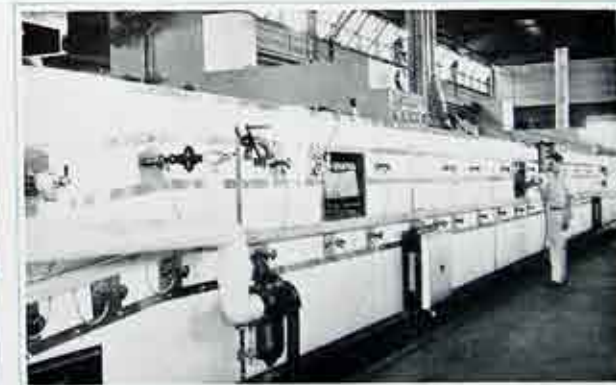
Some of the varied activities of the Industrial Sales Department are reflected in the above illustrations: Top, modern lighting installation at the Davenport Machine Tool Company; center, new kitchen at the new Masonic Temple; and, bottom, 92-foot Baker-Perkins conveyor belt now installed at the General Baking Company's plants.
