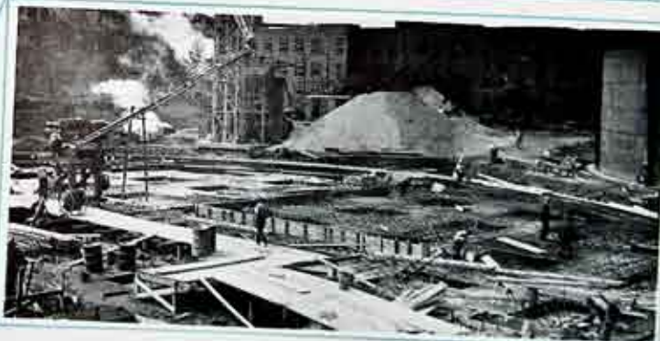
Construction activities, top, progress of work of installing new gas lines at East Station in connection with the new holder; center, building the foundations for the new Koppers oven; at West Station, and, bottom, building the foundation of the new holder in which a concrete bed 27.5 inches thick and the largest yet used in construction circles, was supported on 87 piers sunk to bed rock.
