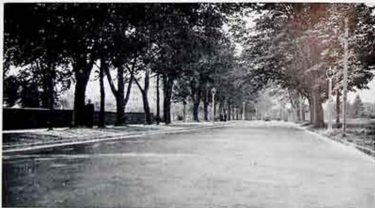
A total of 1,556 underground-fed lamps were installed last year as well as 157 of the overhead-fed type. Shown above is a section of Lake Avenue Boulevard where between Winchester Street and the B., R. and P. Railway bridge forty-five 400-candlepower lamps were installed on concrete standards.
