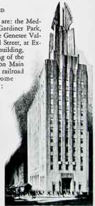
The Genesee Valley Trust Company, on Broad Street, which is to be heated with Company steam.
