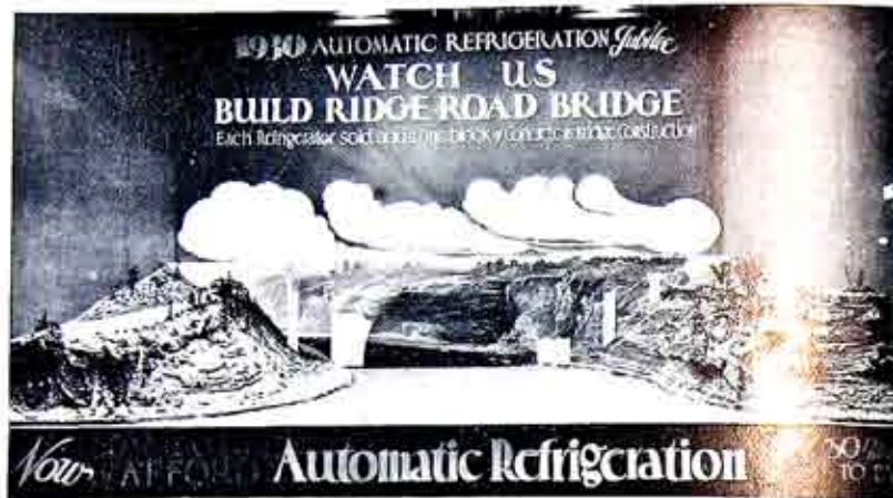
This is the window that commanded attention. Ridge Road Bridge a few days after construction began.
