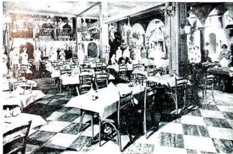
The lighting of Old Spain was so planned that there may be obtained by the mere manipulation of switches, the sunny aspect of noonday, dusk tones, or the more subdued lights of sunset. Lighting is direct, indirect and semi-indirect and the wiring and outlets are sufficiently adequate to permit almost any desired combination of illumination at will.
