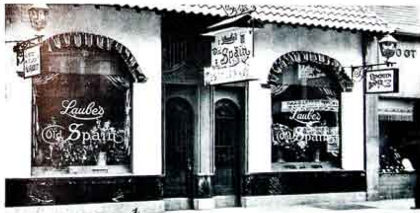
Old Spain Restaurant, of the Laube Chain of restaurants, which recently opened its doors to the public at 11 East Avenue, Rochester. Over $3,500, represents the Company's sale of modern kitchen and restaurant equipment for this eatery which, inside and out, breathes the atmosphere of Sunny Spain.
