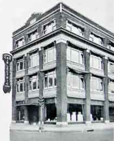
Main office building at Cornell and Green Streets.
