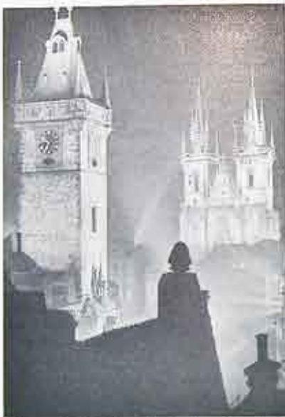
Old City Hall, Praha, Czechoslovakia, showing in distance Hussite Church, built in the Fourteenth Century. Photo used by courtesy of Mr. Pergler, who visited our company some months ago.
