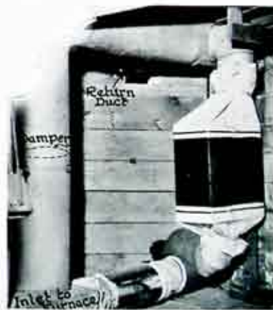
Details of Mr. Taylor's installation, from which he obtained some interesting data bearing upon home ventilation.
