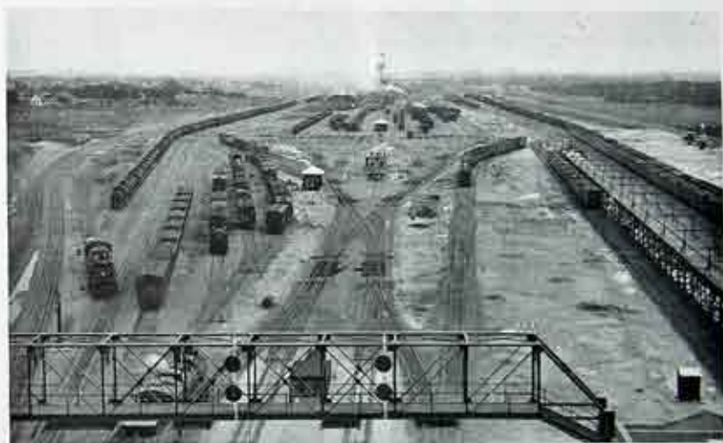
Lancaster Hump Classification Yard at Ft. Worth, Texas, on the Texas and Pacific Railway. Car by car, trains hauled up the inclined tracks in the center of the illustration, aided by gravity speed down the incline again and, controlled by G-R-S car retarders, safely and quickly are shunted to the particular track desired, saving hours of old-time switching, with its pulling and hauling, car riders and added expense.
