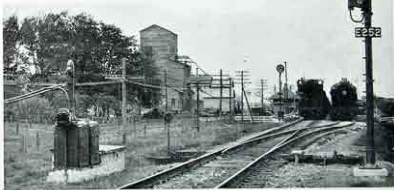
Signal location in the G-R-S Dispatching System of the Ohio Division of the New York Central Railroad. The view shows how the dispatcher, by means of these signals, has passed one train around the other.
