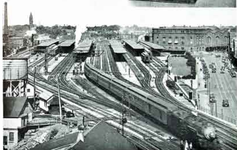
Top, G-R-S Interlocking Machine used to operate the switches and signals at the Rochester Central Station. Below, general view of the Rochester Station which is fully equipped with the G-R-S System of Electric Interlocking. The operator at the machine above controls the movements of all trains entering, passing through and leaving the station by means of these electrically controlled devices.
