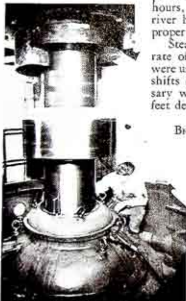
Shaft of New Turbine at Station Five.
