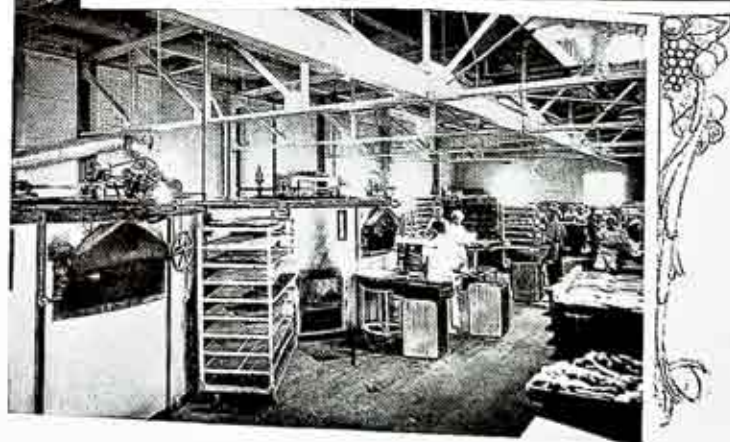
Top, electrical refrigeration installation at the Rochester Park Market; center, Baker-Perkins gas fired wafer oven at the plant of the Beecham Packing Company; bottom, scene in the Weble Bakery, where all three of the Company's chief products, gas, electricity and steam are utilized.
