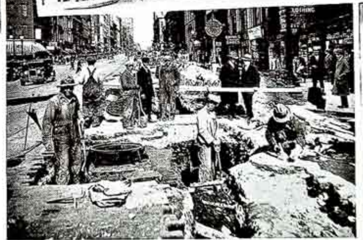
Top, Barge Canal Harbor, and new Court Street Dam in operation; middle, the new lighting on Main Street East and, bottom, how the Company took advantage of the opportunity to enlarge manholes and increase its ducts during the widening and repairing of Main Street.
