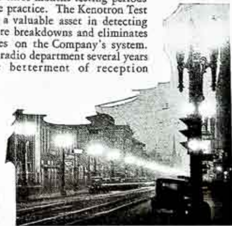
North Street's new lights as viewed at dusk from the corner of North and Andrews Streets.
