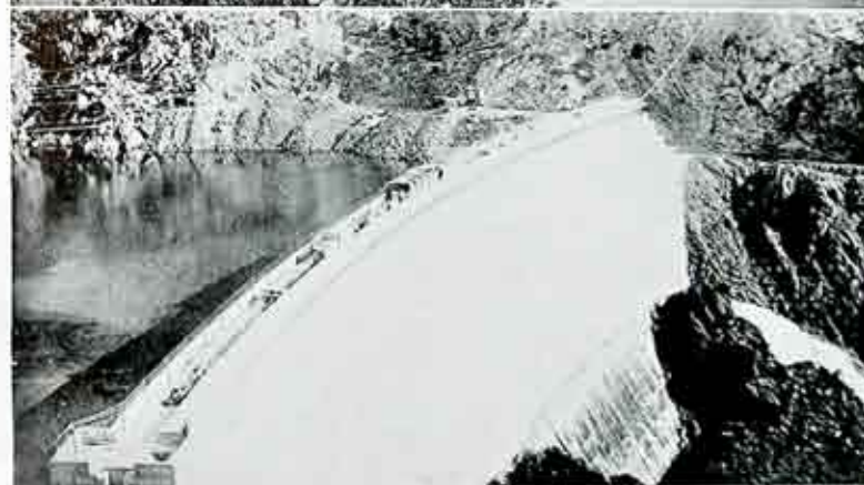
Top: Cotter River Dam, Canberra, Australia. Middle and Bottom: Burrinjuck Dam, Province of New South Wales, which is 250 feet high, 752 feet long and holds 34,000,000 cubic feet of water.
