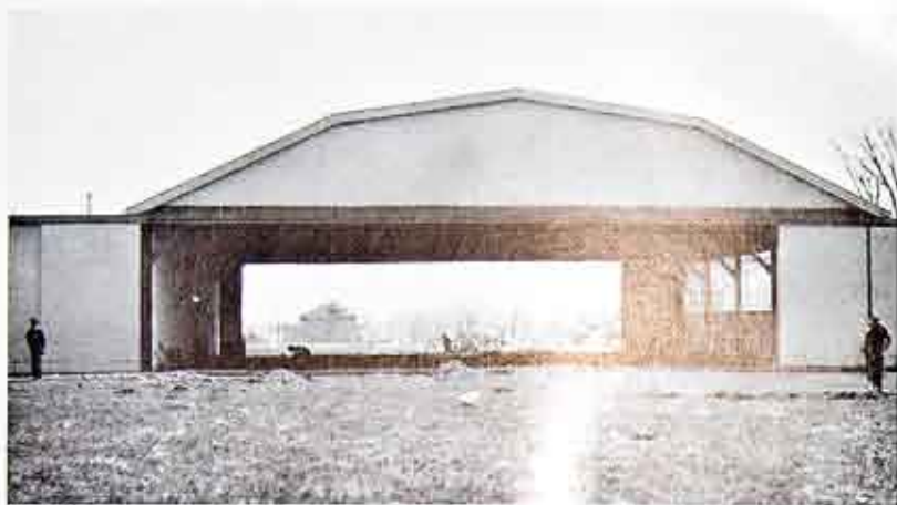
Rochester Airport Hangar. The hangar is built according to the latest government specifications and makes a fine haven for municipal visiting ships.
