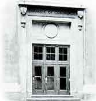
The main entrance to the Rochester Chamber of Commerce on St. Paul Street.
