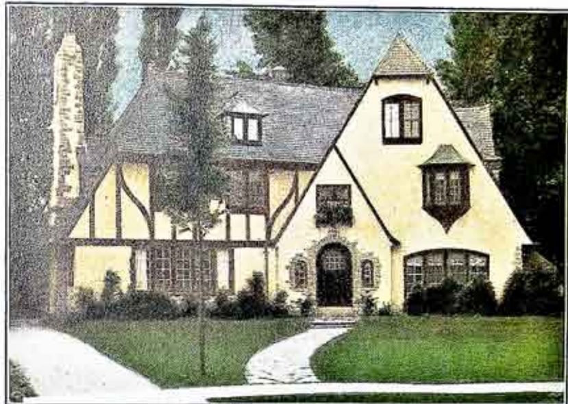
Home of Mr. Clarence Wheeler, 57 Dorchester Road, which is heated by a gas-fired hot water system. This is one of the many Rochester gas-heated homes, featured at the Company's exhibit, in colored transparencies, at the recent Rochester Industrial Exposition.
