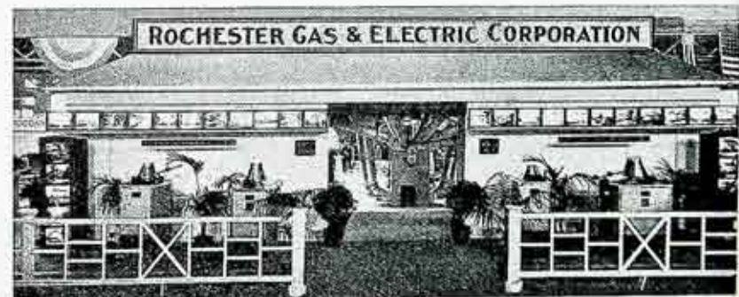
North side of the Company's Exposition exhibit which illustrated graphically and in detail some of the advantages accruing from heating homes by gas. Thirty-two colored transparencies of Rochester gas-heated homes were featured in this portion of the exhibit.
