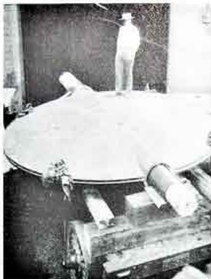
Figure 4. Mr. William Claire standing on 25-ton butterfly valve which was installed in No. 3 penstock shown in Figure 3.
