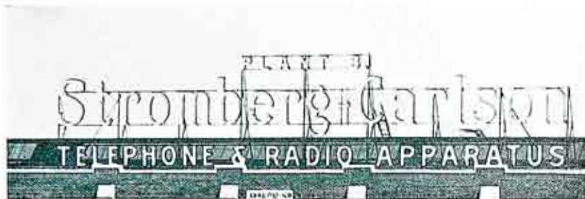
Attractive electric sign installed by the Company on the new plant of the Stromberg-Carlson Company on University Avenue.
