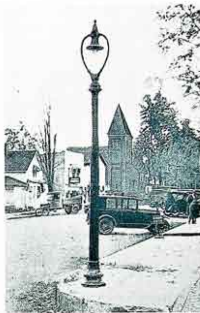
One of the 15 Class S, 400-candle power lamps recently installed in the downtown section of Pittsford, on ornamental metal standards.
