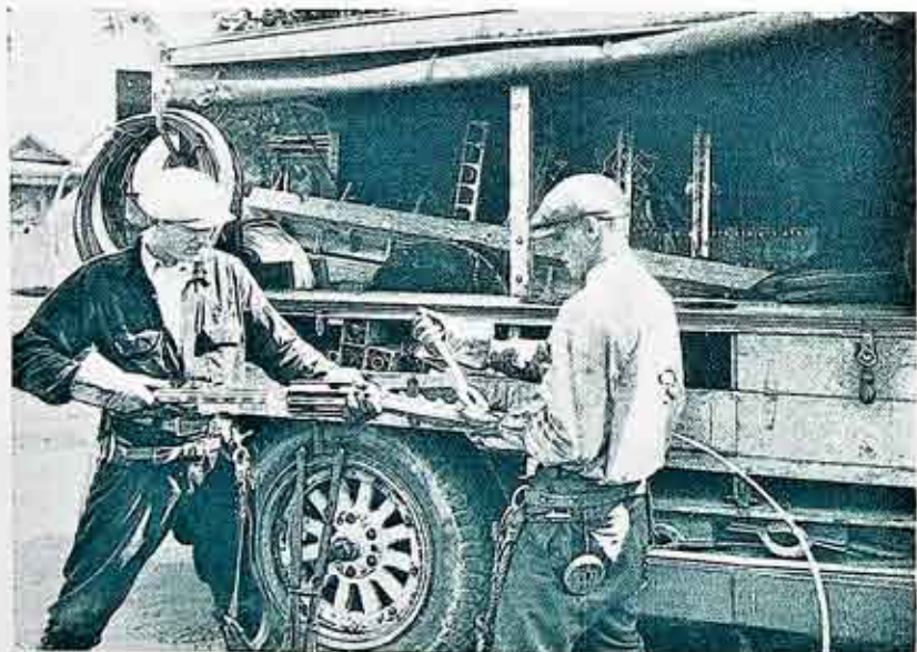
Line trucks are equipped with sufficient materials to make possible emergency installations. These linemen, Messrs. William Shears and Roy Mahey, are making up the anchor guy illustrated on the last page of this article.
