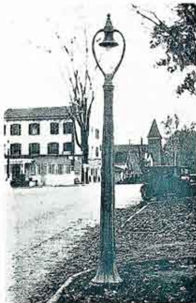
One of Pittsford's 77 new Class O, 200-candle power lamps, mounted on concrete standards. The concrete poles were used in the residential district.
