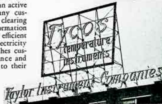
New electric sign installed by the Domestic Sales Department on the top of the Taylor Instrument Plant. This attractive sign is easily visible to night or day travelers over the N. Y. C. Railroad's Main Line.
