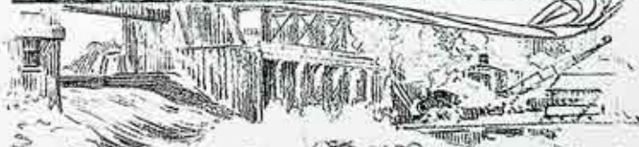
Construction work at the Court Street dam comprises the addition of two 110-foot sections of movable sector gate dam to replace the section of Mohawk dam formerly operated there in conjunction with the two 55-foot sections of State sector dam, which will remain intact.
