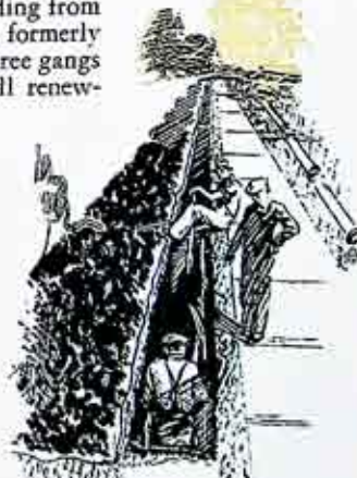
Over 40 miles of gas mains were installed during 1926.
