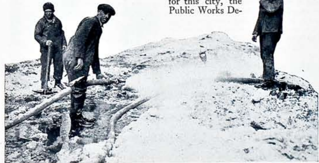
Fig. 2: The Use of Fire Hose to Disintegrate Snow Banks is Very Effective
