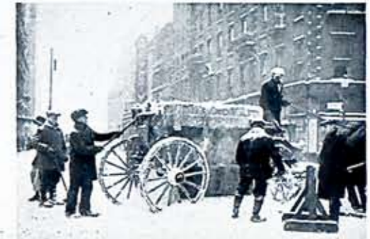
Fig. 1: Dumping Snow into the Tunnel at Fitzhugh Street
