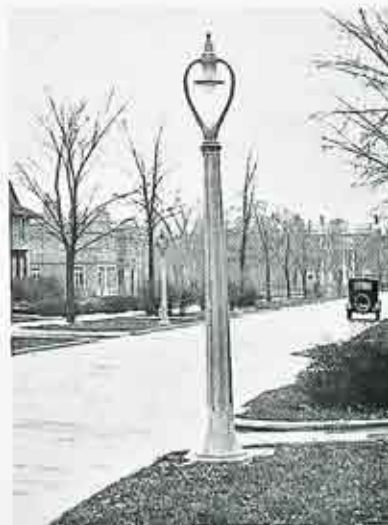
In Rochester Underground Wires Make Safe and Beautiful Streets Possible.
