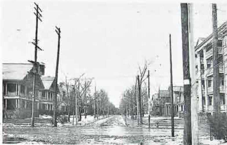
Most of Toronto's Street Lamps are Attached to its Wooden Poles. Would Rochester Citizens be Satisfied with this Arrangement?—We don't think so.
