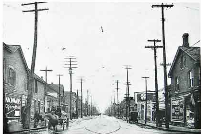
Dundas Street, Toronto, where 2 Lines of Trolley Poles, 1 Line of Telephone Poles and 4 Lines of "Hydro" Poles add Nothing to Appearance and Comprise a real Safety Hazard as well as a Source of Service Interruption.
